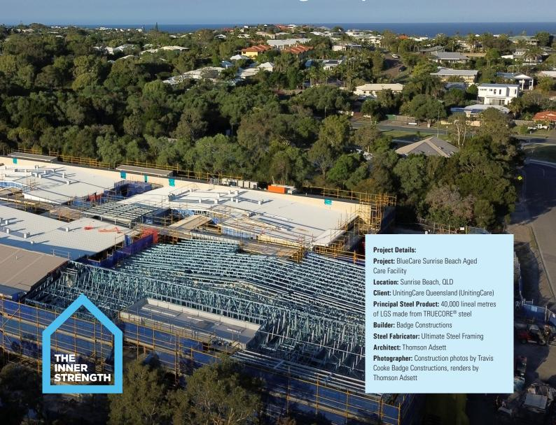
Designed and prefabricated off-site, light gauge steel (LGS) framing made from TRUECORE® steel allows a critical aged care facility to be built on schedule and on budget.
