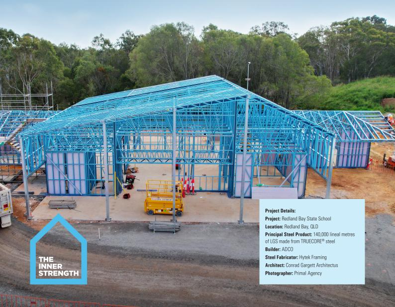
Lightweight and strong, light gauge steel (LGS) framing made from TRUECORE® steel is designed and prefabricated off-site, requiring early collaboration between builder, engineer and fabricator.
