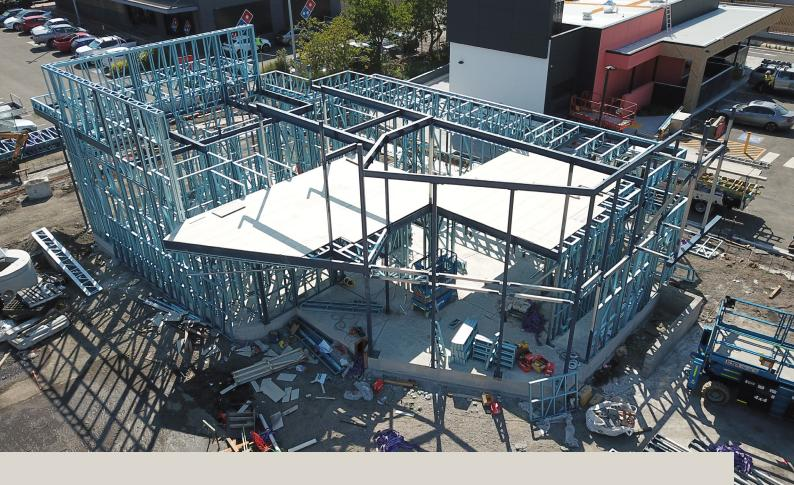
Building Information Modeling (BIM) ensured the benefits of using light gauge steel (LGS) framing made from TRUECORE® steel expedited the project timeline of this Illawarra fast food outlet.
