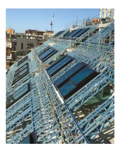
securely connected to these slabs using a method that allowed for slab deflections. The final facade structure was also designed so the battens could be appropriately installed at defined intervals to support the roof tiles.
