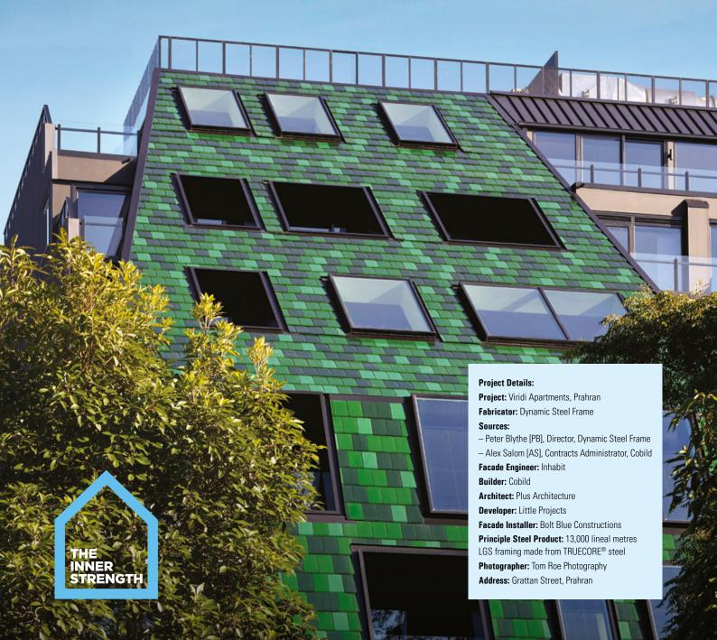
Lightweight yet strong, light gauge steel (LGS) structural framing made from TRUECORE® steel was the material of choice for the striking facade structure inspired by its parkland surroundings.
