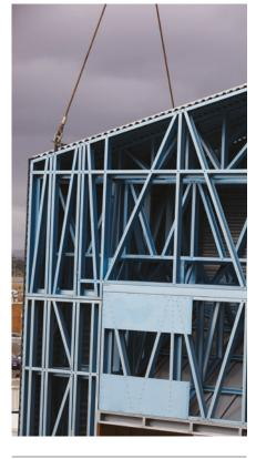
Utilising approximately 3km of TRUECORE® steel and weighing close to 7.2 tonnes once the external cladding was installed, the lightweight yet strong framing managed the stress of the crane lift without damaging the cladding material.
