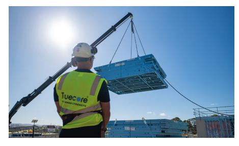
enhance labour efficiency, even on restricted sites with multiple townhouses and duplexes. Site management is also improved by the big reduction in onsite waste that comes from building with frames made from TRUECORE® steel.
