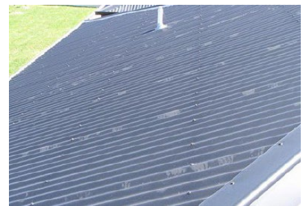
Figure 2. Roofing with sunscreen damage
