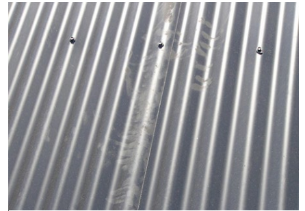
Figure 2. Roofing with sunscreen damage
