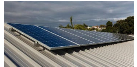
Figure 1. An example of a framed PV panel mounted above a steel roof
