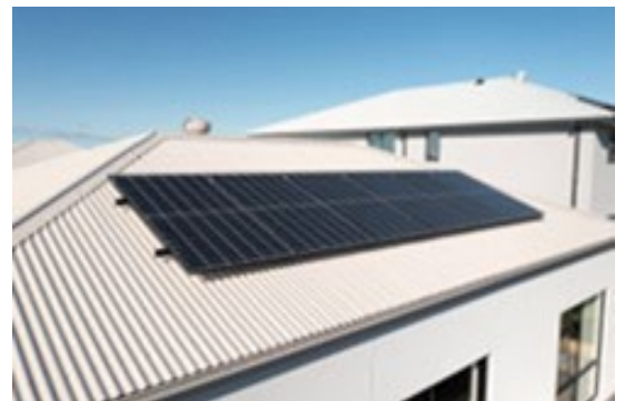
Figure 1. An example of a framed PV panel mounted above a steel roof
