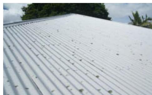
**Figure 5. Roof made from COLORBOND® steel showing uniform coverage of fungus**
