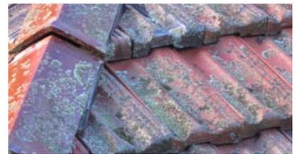
**Figure 2. A close up of a) fungal and b) lichenous growth**
