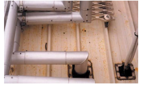
Figure 1. Swarf staining
