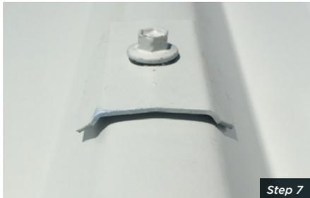
**8** Barge capping needs to accommodate the slight rise in the joint area.
