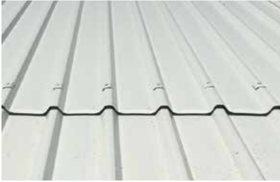
Completed lap joint
