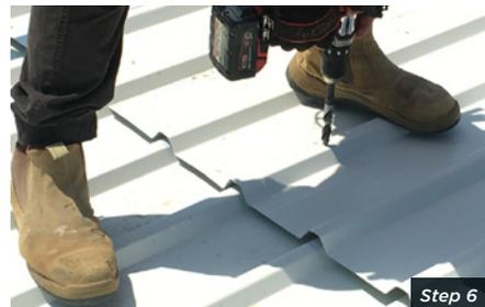
**7** Position a MonoLap® cap over the 16mm diameter hole. Screw through using a No 12-14x68mm tek screw through both layers of sheeting and into the support below.
