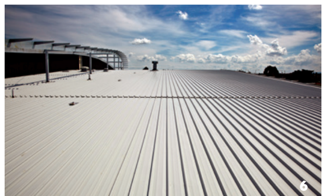
Completed lap joint
