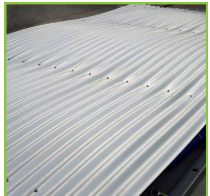
Roof Pressure Test
