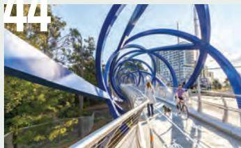
The Christopher Cassaniti Bridge is Australia's first double-helix bridge and provides the connection between the residential Lachlan Line's development to North Ryde Metro Station, spanning the M2 Motorway and Delhi Road without interruption to traffic.
