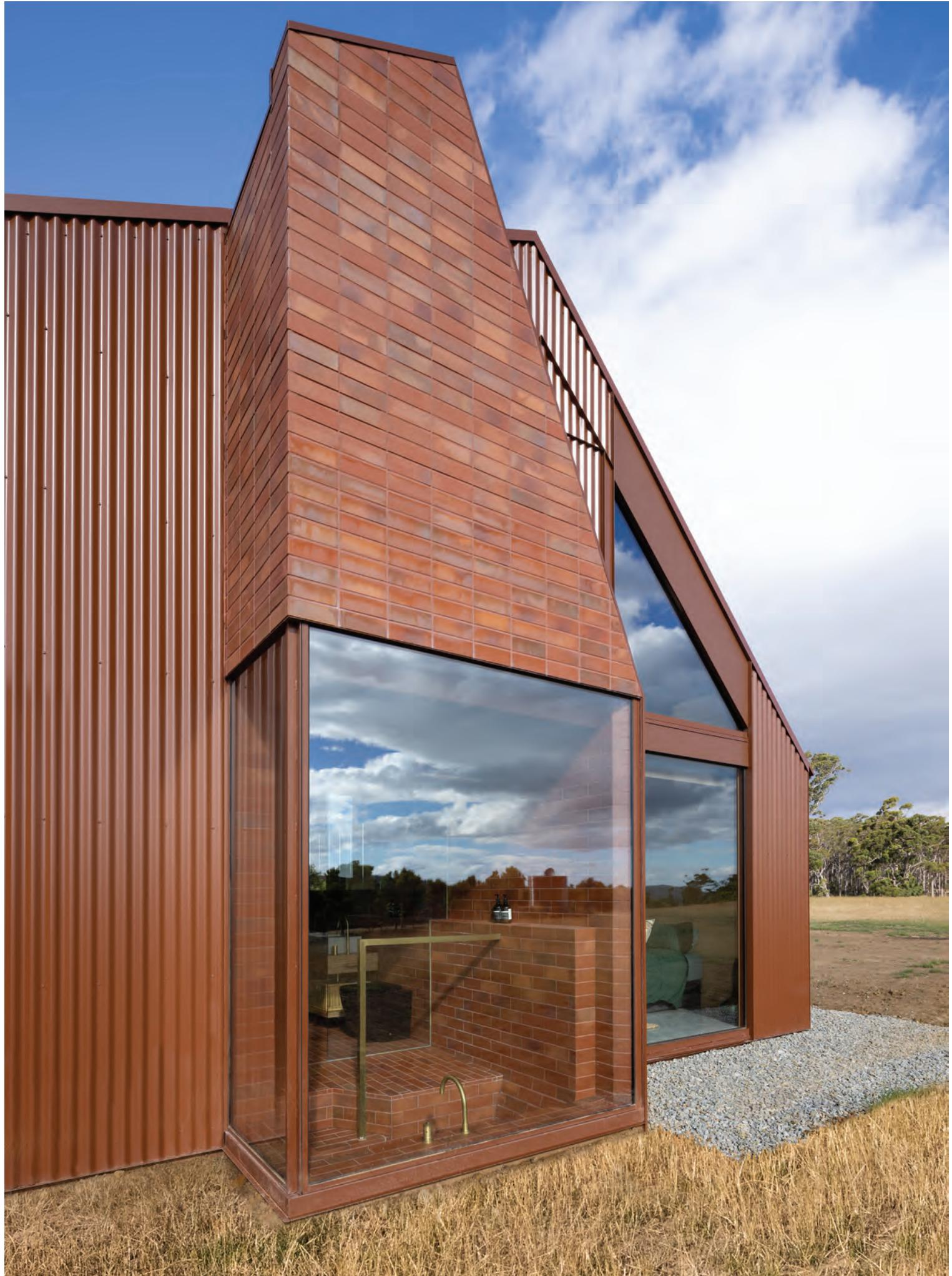
“We used COLORBOND® steel because it’s lightweight, easy to transport, highly durable, easy to install and the colour is a strong reference and direct connection to the existing red-lead shacks on the island. It was always going to be steel”
