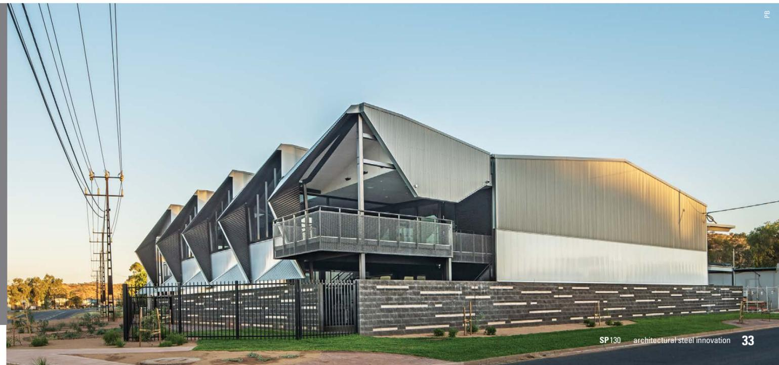
The main shed walls are made from COLORBOND® steel in LYSAGHT CUSTOM ORB® profile, in the colour Windspray®, matching the cladding of the sunhoods.
