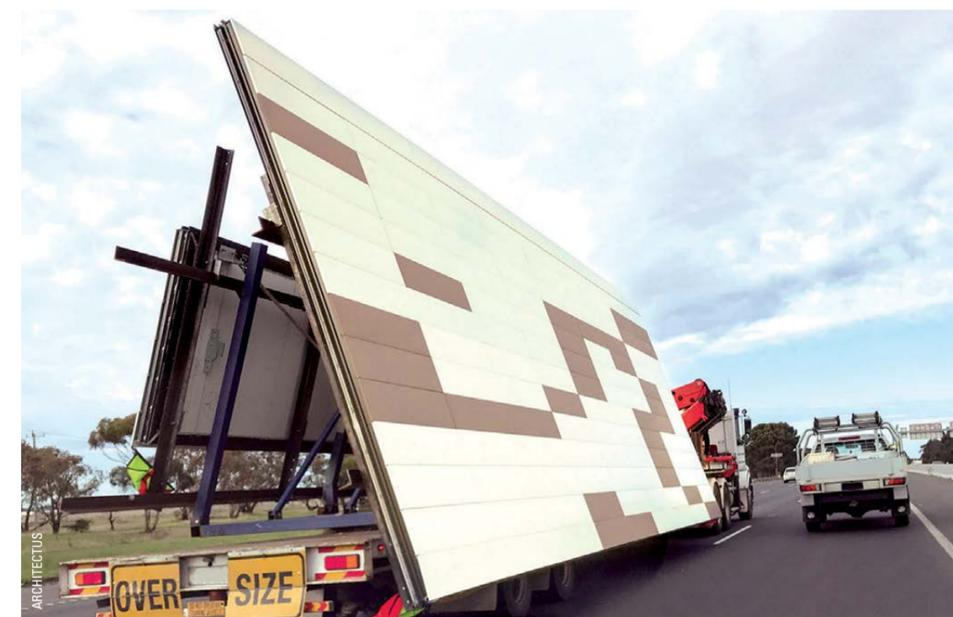
ABOVE: The panel system consists of an exterior rainscreen made from COLORBOND® steel which is fixed to steel sheeting that sandwiches a non-combustible insulation layer. The entire panel is fixed into a rectangular steel portal-frame that runs around its perimeter and the panels ‘clip’ together using a weatherproof mating system.
