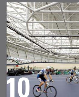
Cox Architecture's design for Queensland's first enclosed cycling track employs 1200 tonnes of steel in an efficient engineering solution for its vast and graceful, saddle-shaped roof structure.
