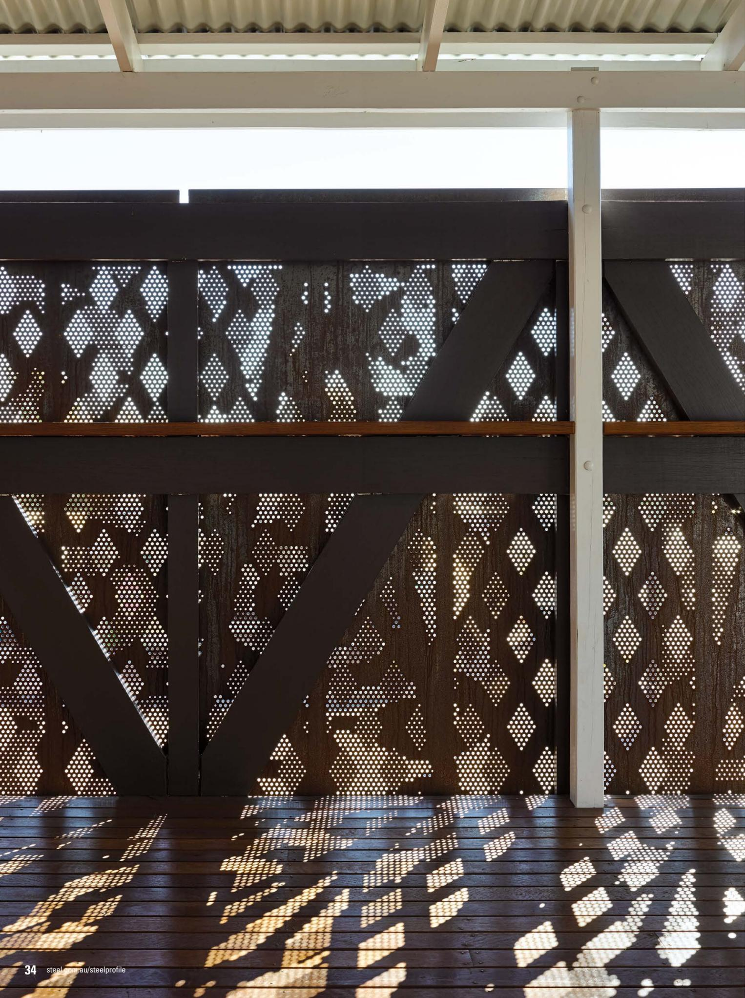
OPPOSITE: The panels made from REDCOR® weathering steel create a winning shade-ventilation combination for the harsh outback environment.
