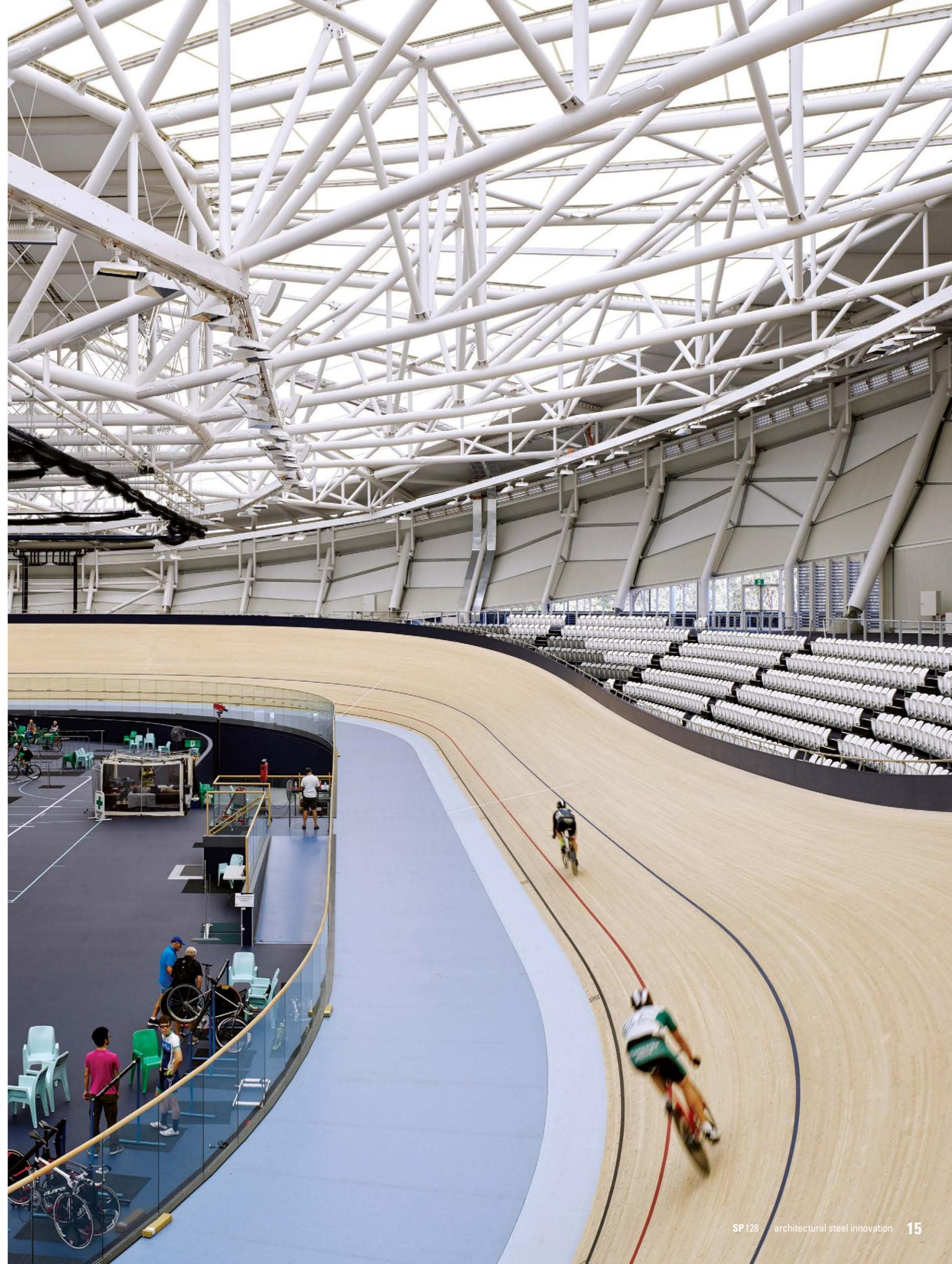
"We chose to use fillet-welded saddle plates on site rather than bolted splices. This meant that major elements of the roof structure could be lifted in, positioned on welded saddle connections and fillet-welded, providing flexibility in terms of tolerances.
