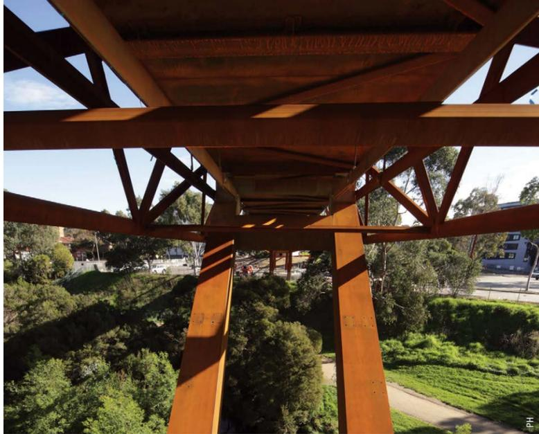
ABOVE: The underside of the bridge resembles a seamlessly integrated structure and platform, thanks to the 'baking trays' – made from 3mm-thick REDCOR® steel coil in 1594 HW350 grade – that provide permanent formwork for the concrete deck.
