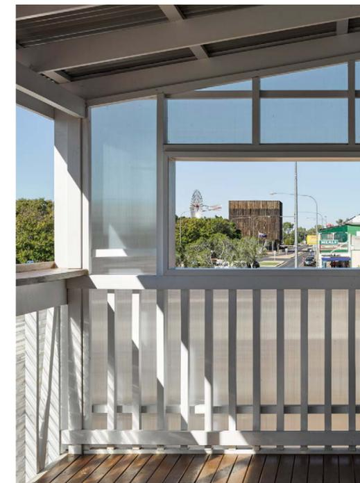
LEFT: Roofing and guttering made from COLORBOND® steel in the colour Surfsmist® was designed and fabricated to integrate neatly with the flashings and polycarbonate screens.
