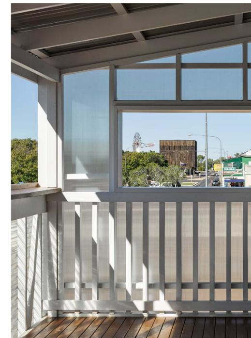
LEFT: Roofing and gutting made from COLORBOND® steel in the colour Surfsmist® was designed and fabricated to integrate neatly with the flashings and polycarbonate screens.
