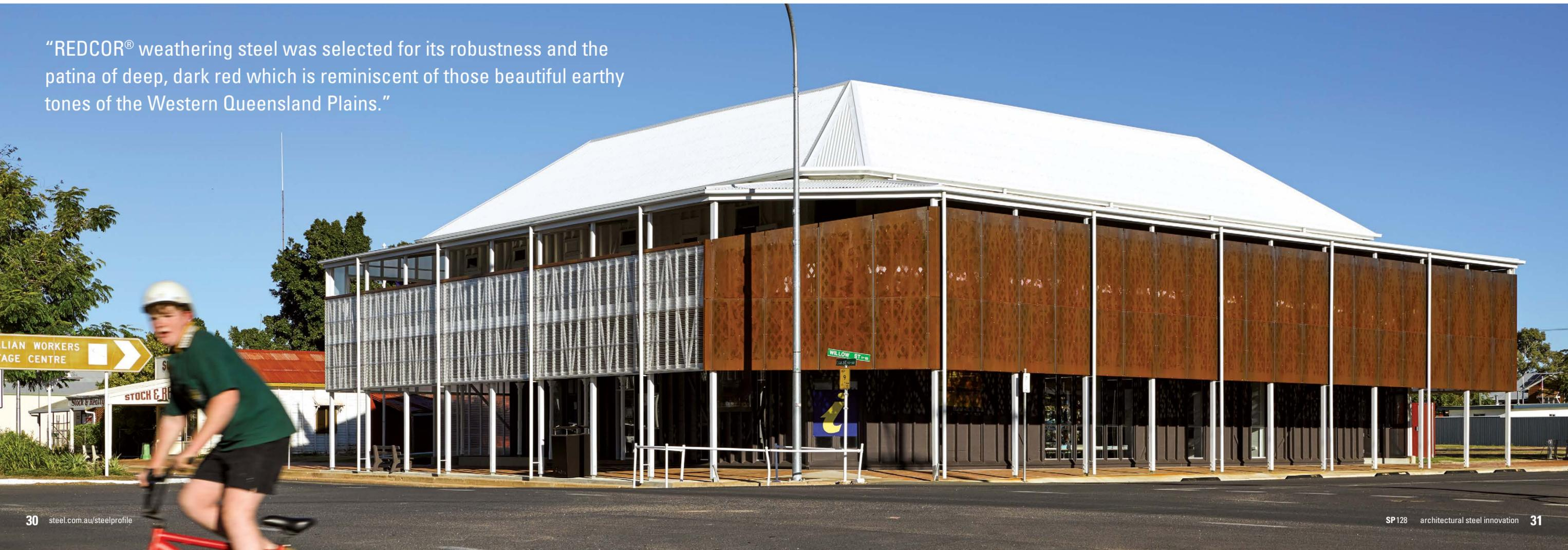
“For its ability to reflect heat and minimise the amount of energy that surfaces such as a roof absorb in an outback environment, a roof made from COLORBOND® steel in the colour Surfsmist® is a practical and pragmatic choice.”
