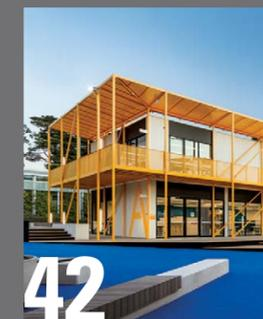
Showcasing steel's slenderness and refinement, Jackson Clement Burrows Architects employed modular prefabrication to drive a rapid program for a temporary building that demonstrates atypical flair.
