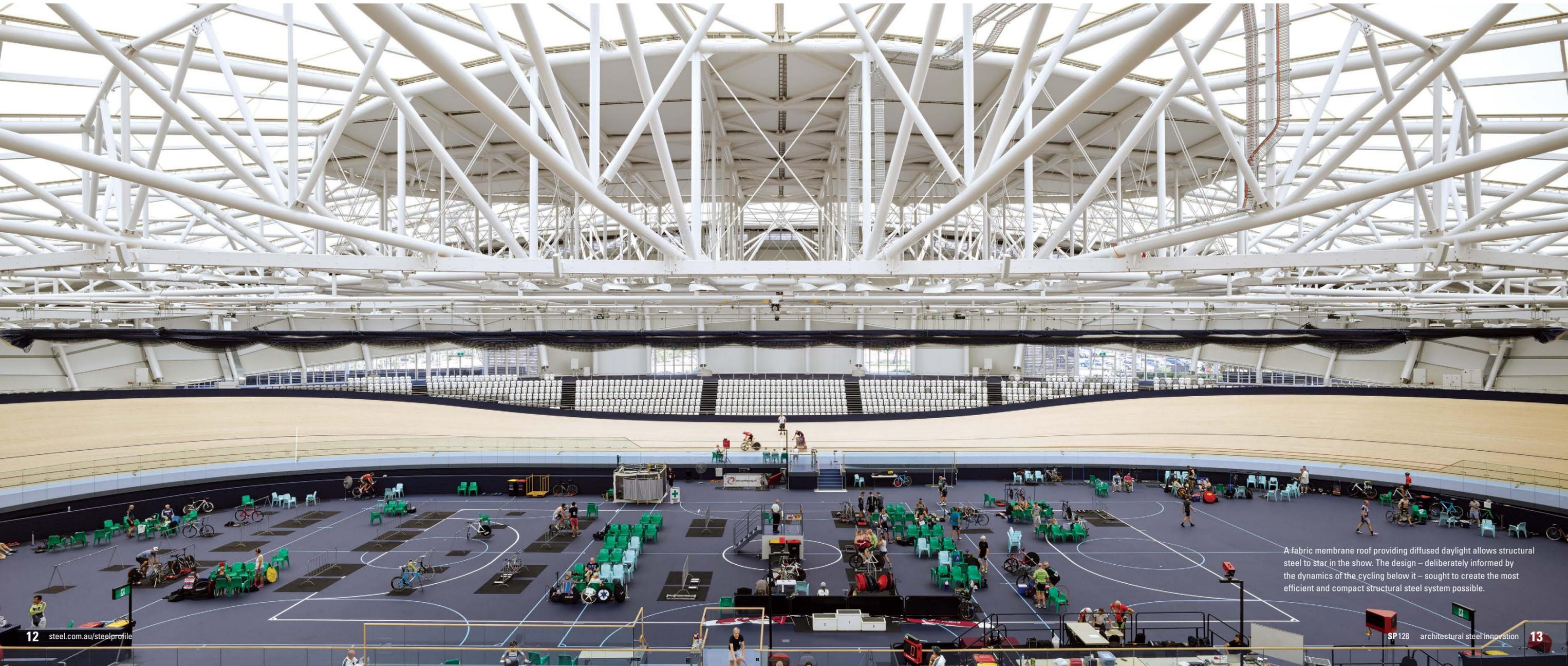
A fabric membrane roof providing diffused daylight allows structural steel to star in the show. The design – deliberately informed by the dynamics of the cycling below it – sought to create the most efficient and compact structural steel system possible.
