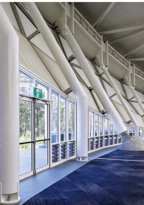
ABOVE: Nine-hundred tonnes of circular hollow sections and 300 tonnes of steel plate, including custom-welded tapering pin joints made from XLERPLATE® steel, were fundamental in achieving the twisting shapes of the saddle-like roof.
