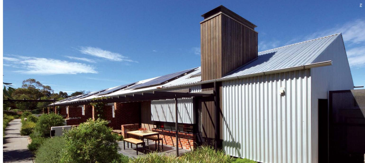
ABOVE AND BELOW: The northern elevation features cladding made from ZINCALUME® steel in LYSAGHT CUSTOM ORB ACCENT® 35 profile as a mediating screen for individual suites, offering privacy and solar control. A simple pergola will eventually be vine-covered to provide dappled shade. The rippled steel surface produces a sun dial effect of moveable shadow and light.
