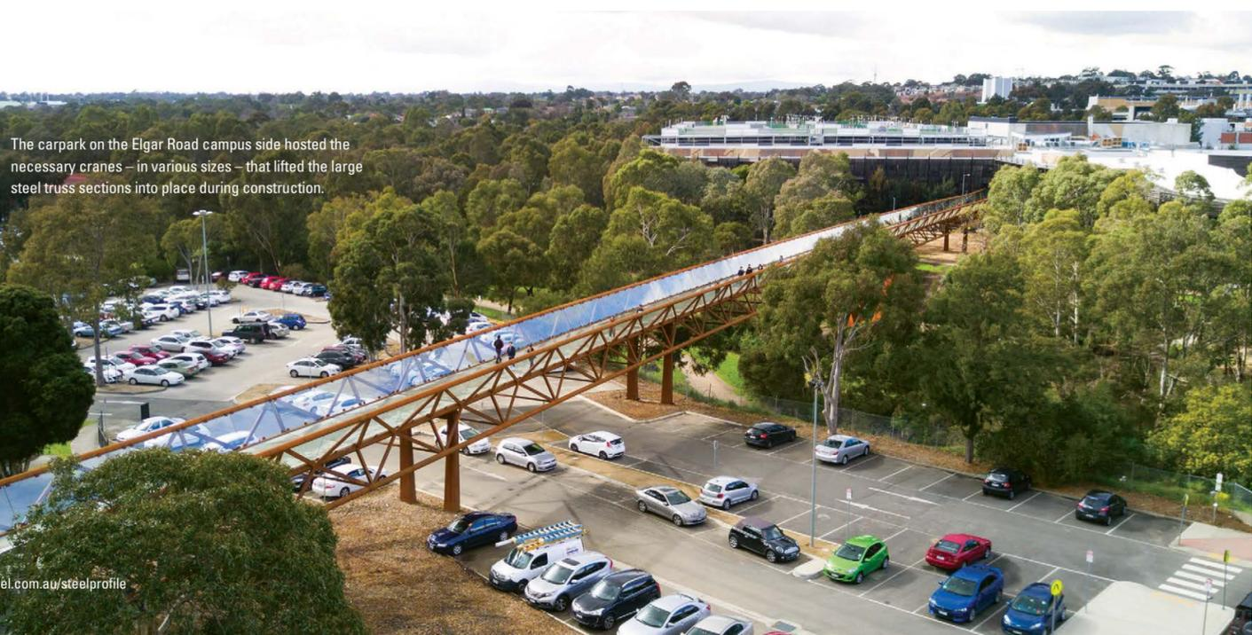
The carpark on the Elgar Road campus side hosted the necessary cranes – in various sizes – that lifted the large steel truss sections into place during construction.
