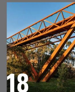
watsonarchitecture+design's inclusion of BlueScope REDCOR® weathering steel to enhance pedestrian access to Deakin University has resulted in a bridge boasting rich, red tones and the unusual ability to both blend in and stand out.
