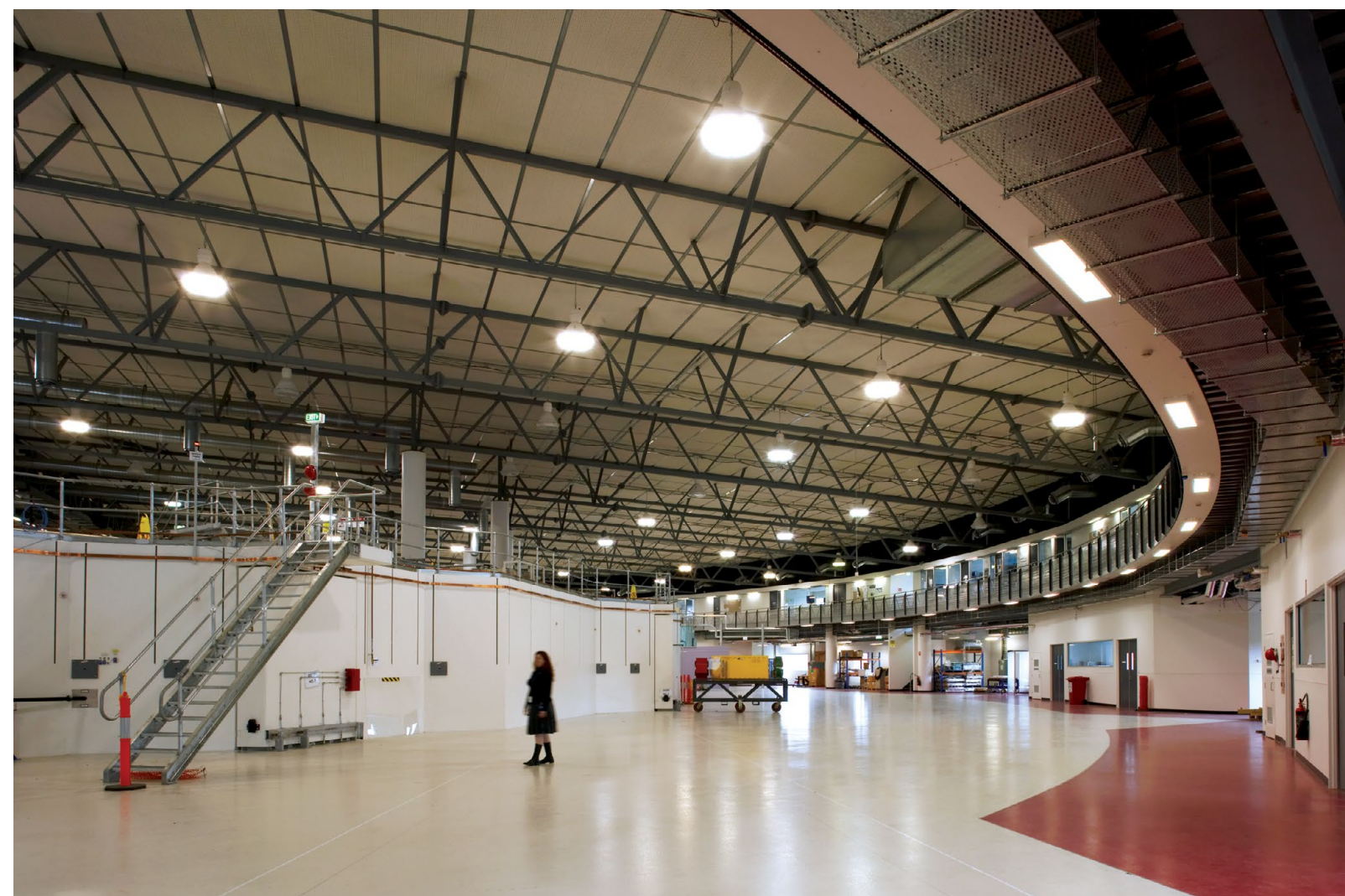
The circular gallery overlooks the heart of the operation, the lead-lined 'machine tunnel', which has concrete walls 800mm thick.
