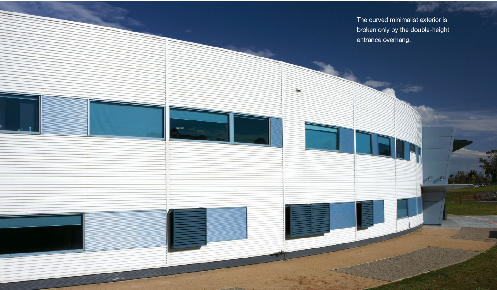
The building presents an impenetrable exterior with windows made from high-performance glass and 12-metre-high walls made from COLORBOND® steel.
