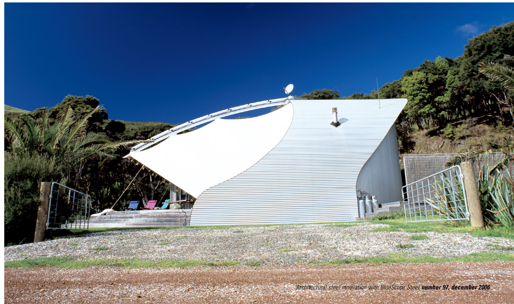
Nestled into the side of a hill, the striking home is dominated by curves, with a white, tensioned membrane stretched over a steel frame juxtaposing the balance of ZINCALUME® steel skins.
