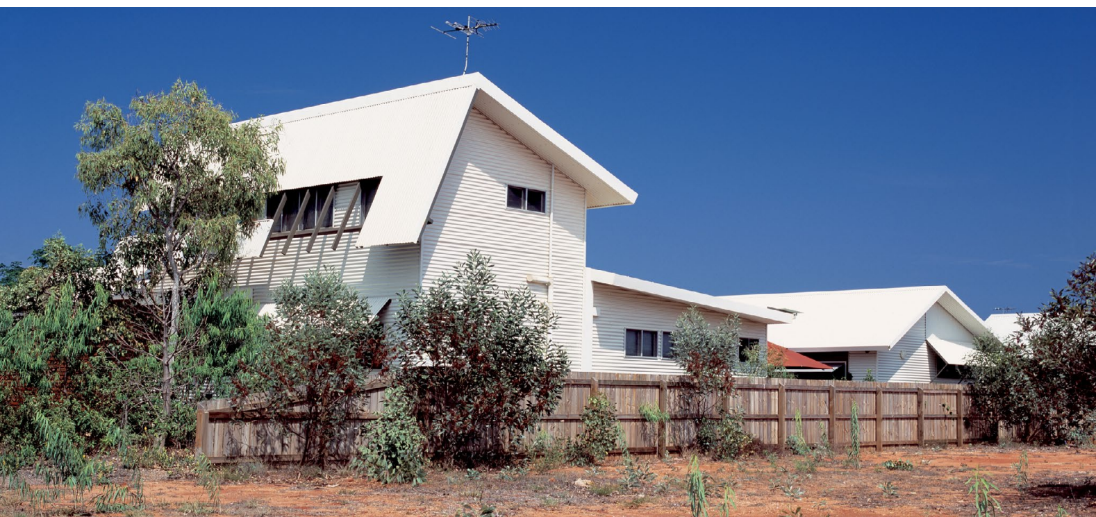
The unusual roof design captures and funnels cooling ocean breezes: a contemporary solution to an age-old climate issue.
