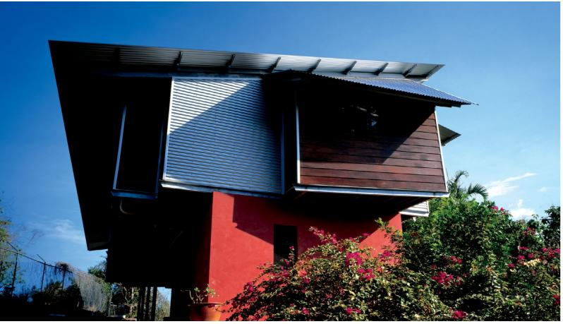
(top) West elevation reveals raking roofline, north-facing balcony and awning as discrete element to help deal with high solar loadings.
