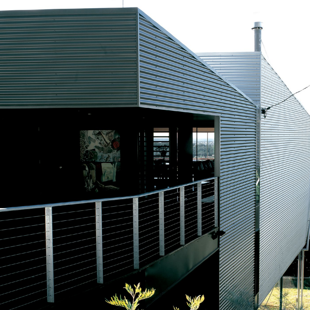
The corrugated steel cladding provides a contemporary look that requires minimum maintenance - a bonus when literally building on a cliff-face.
