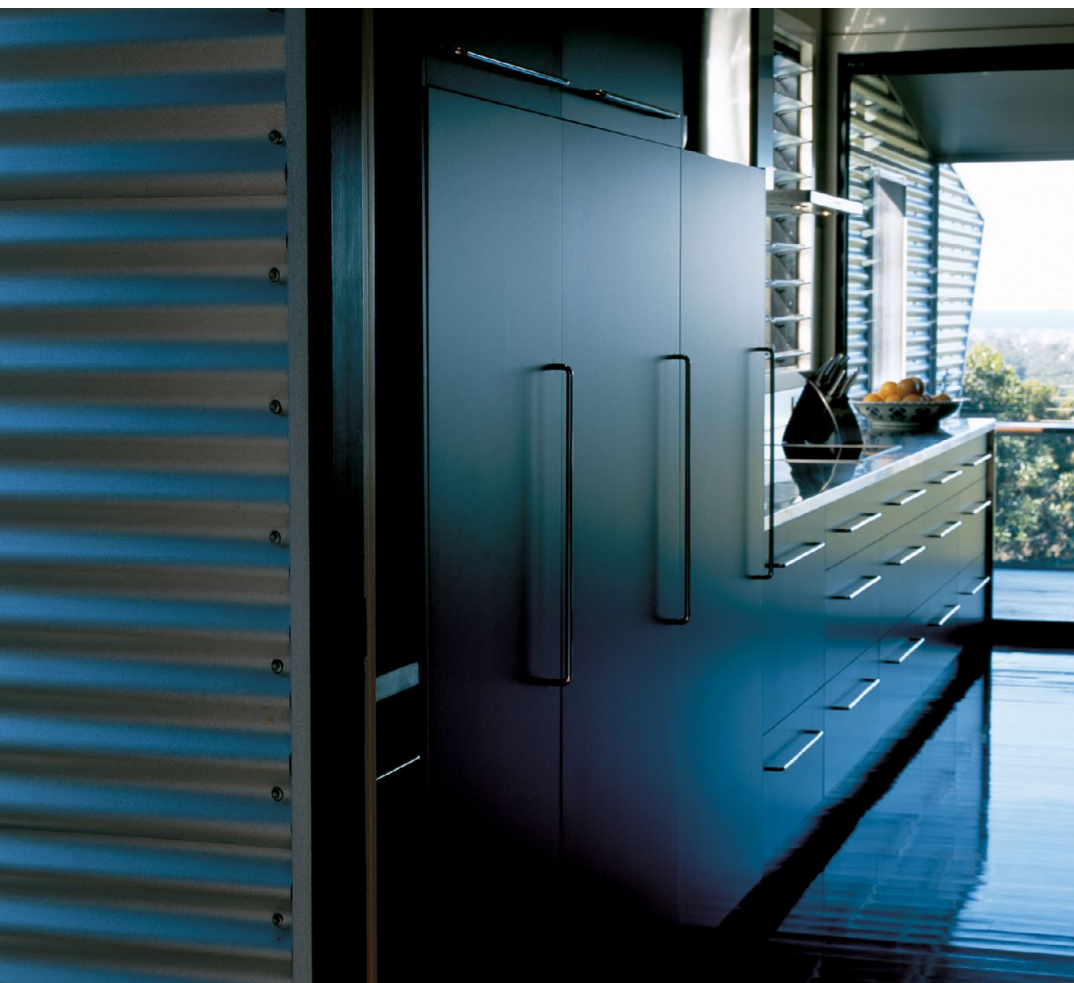
The corrugated steel cladding provides a contemporary look that requires minimum maintenance - a bonus when literally building on a cliff-face.
