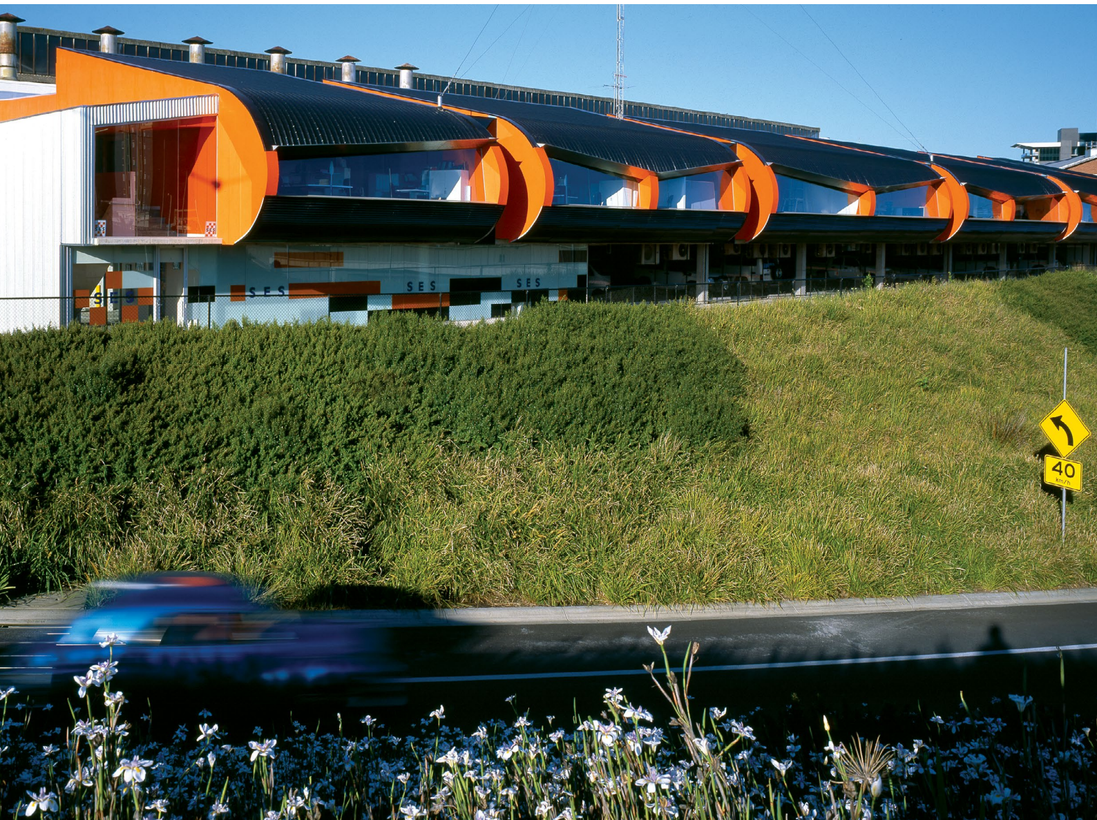
(below) Feeder lane to the Burnley Tunnel entrance offers an exhilarating glimpse of the SES home.
