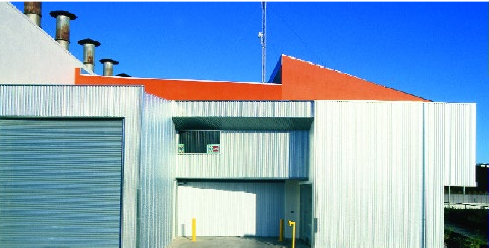
(top) Western elevation provides vehicle service bay and undercover parking.
