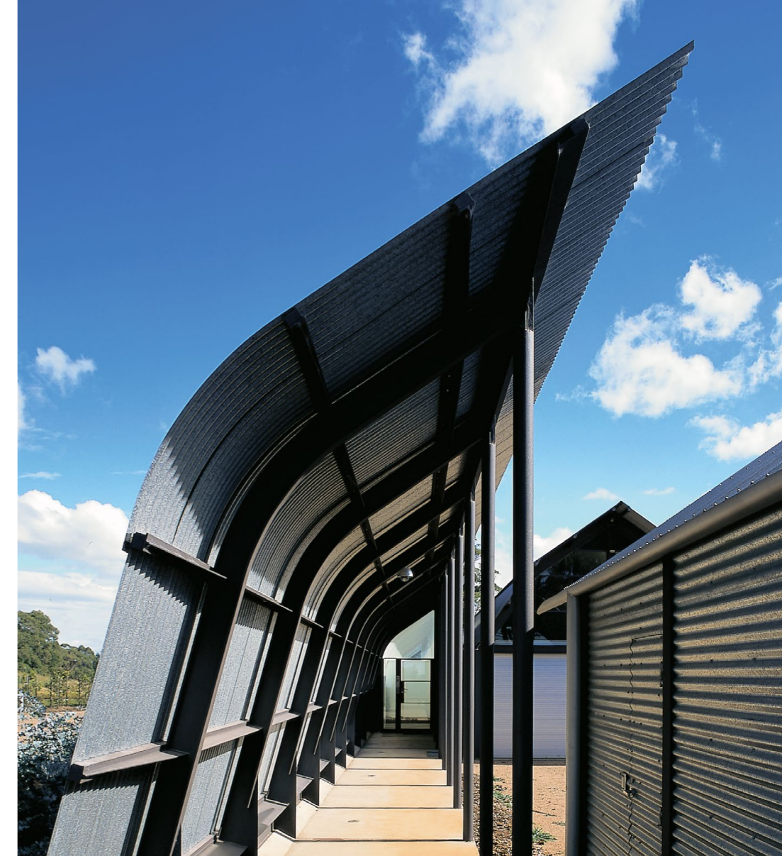
(above and below) Curved corrugated steel kicks the wind from the Southern Alps up and over the house.
