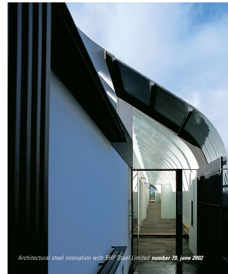
(above and below) Curved corrugated steel kicks the wind from the Southern Alps up and over the house.
