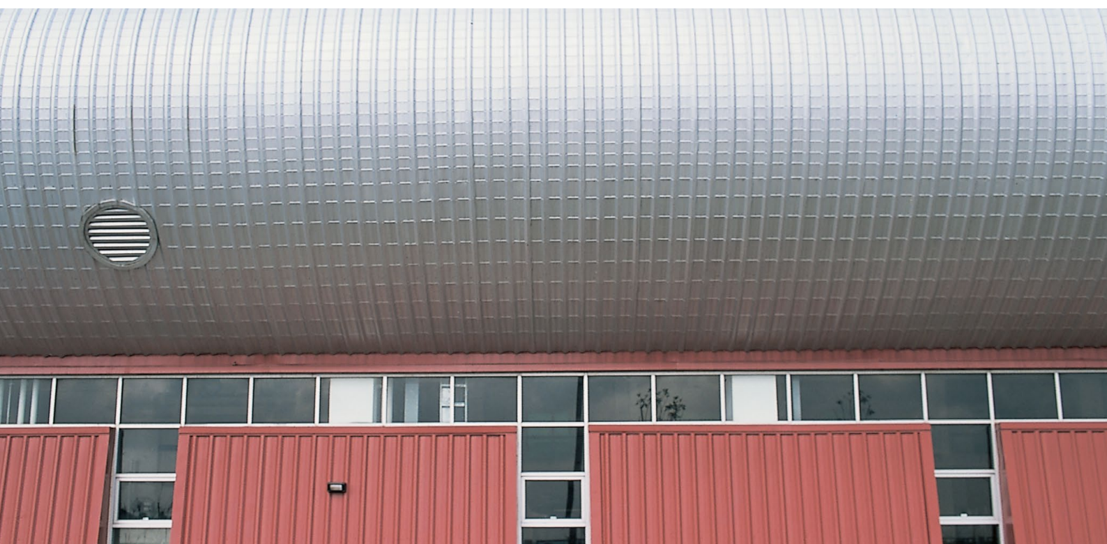
(below) The curved ends of the steel roof form conceal machining and ducting.
