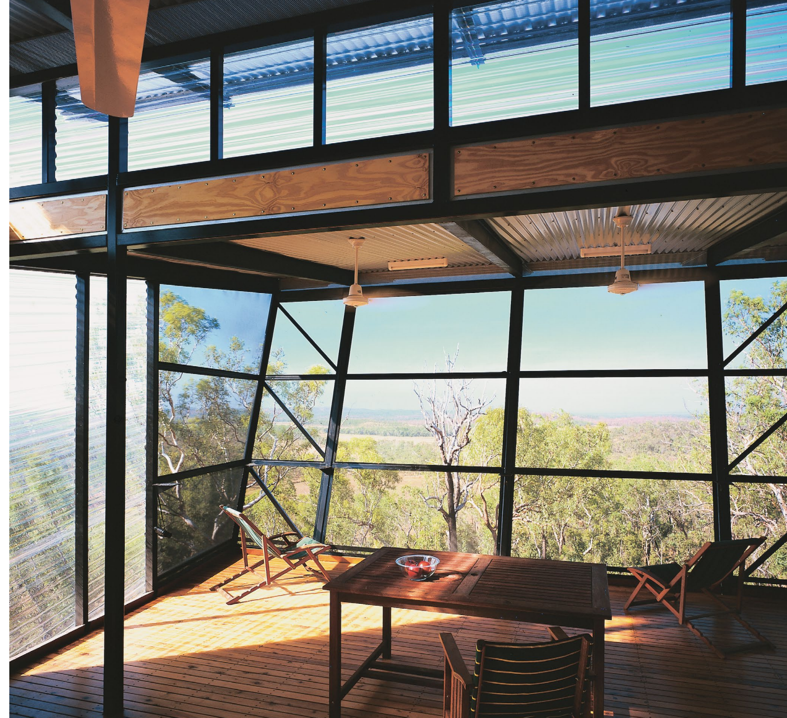
(above and left) Troppo's inside-out theme is aided by lightweight steel construction and an elevation designed to ensure maximum ventilation.
