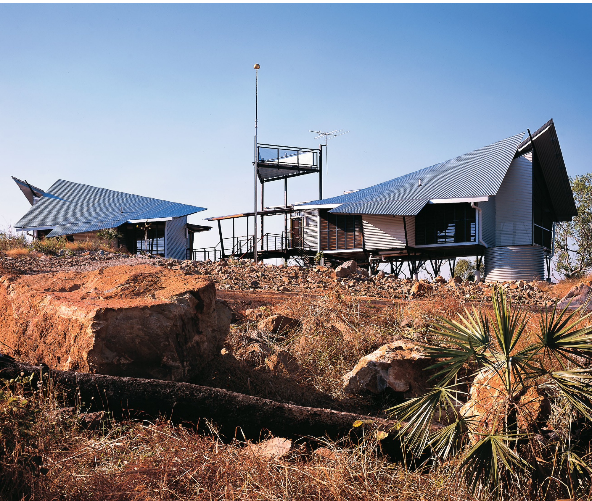
(above) Side wings are linked to a central pavilion whose rear entrance is marked by a steel tower which acts as both a viewing platform and lightning rod.
