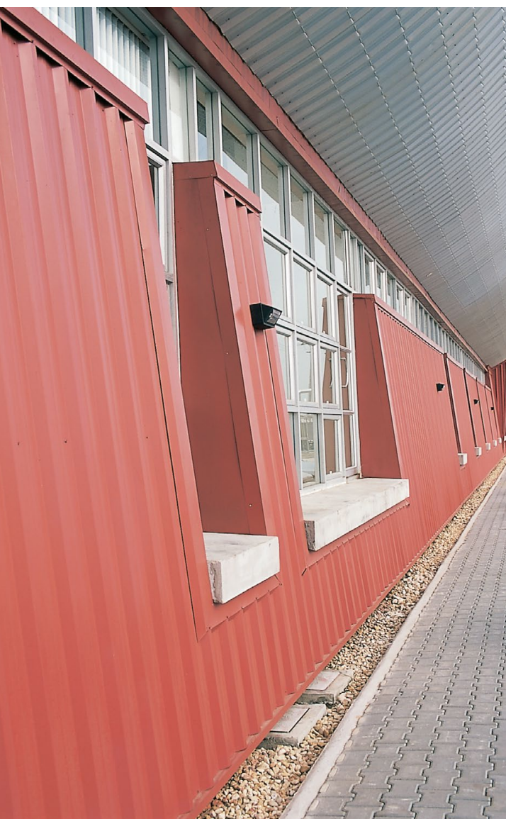
(below) Inclined walls support the "egg" element central to the facility's design.
