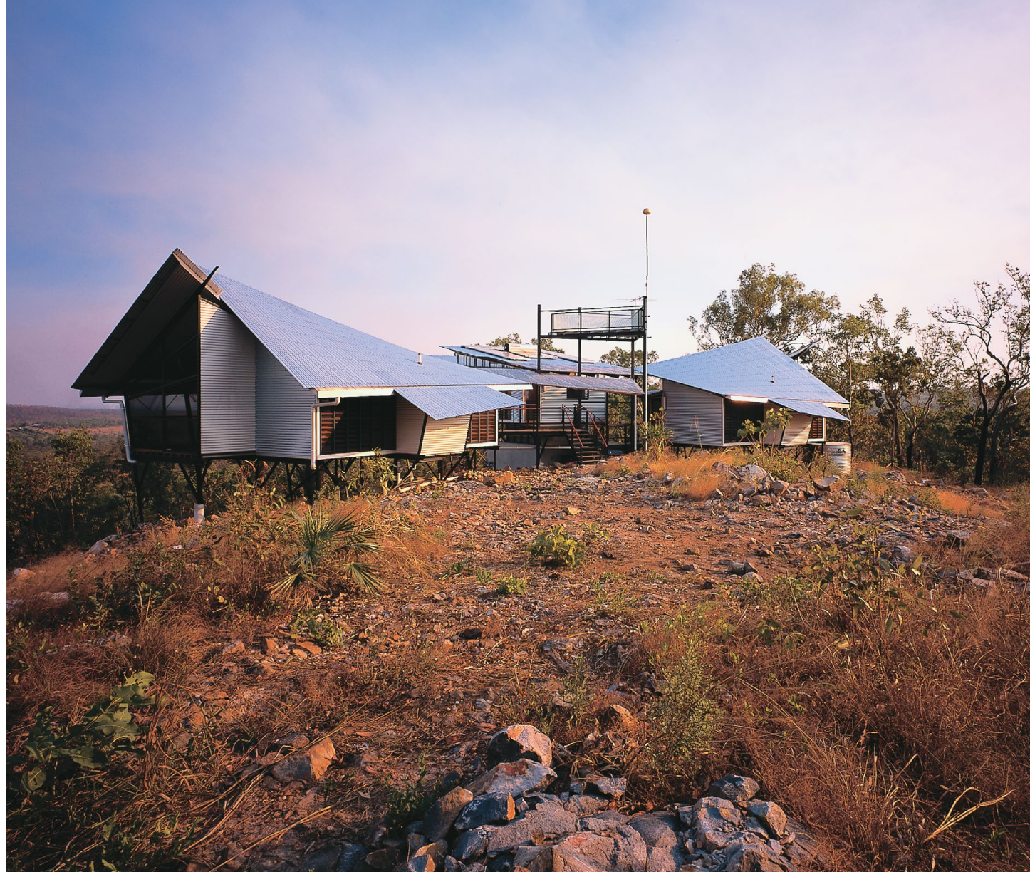
(above) The pitches of the steel roofs are designed to vent hot air by convention.
