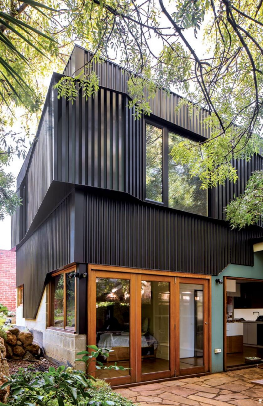
LEFT AND BELOW: COLORBOND® steel in Stramit Longspan® profile, in the colour Nightsky®, wraps sympathetically around the existing timber and concrete-block envelope
