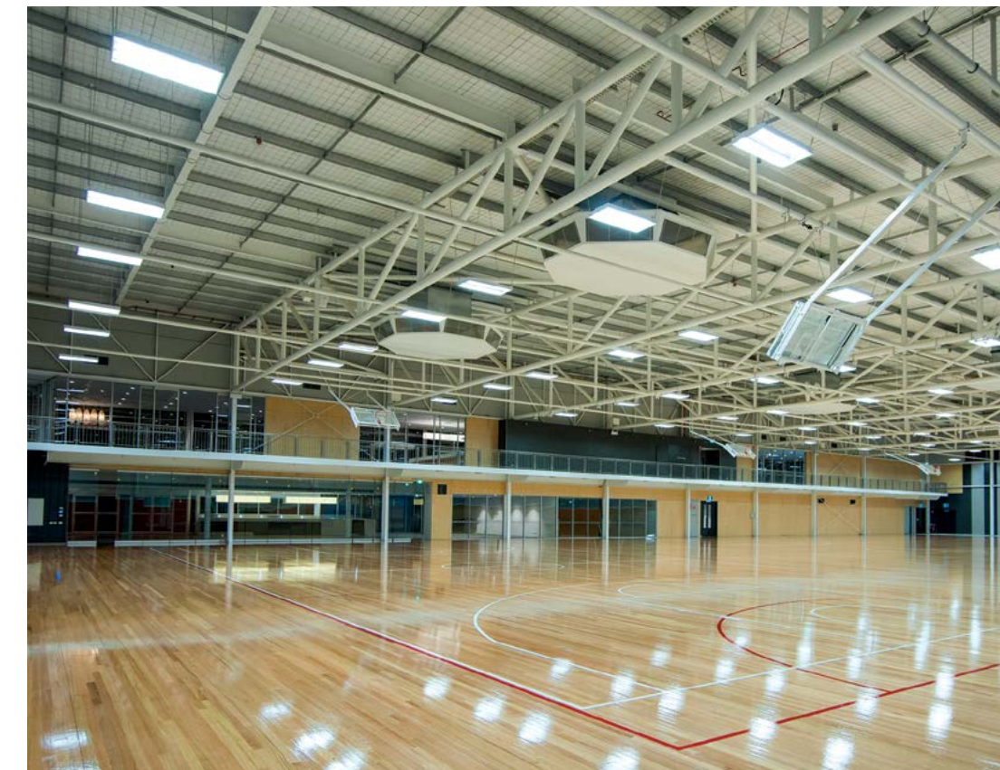
ABOVE: Tubular steel trusses that hang above the basketball courts are as dynamic as the exterior's roof overhang, but also light in form so as not to cause a distraction for spectators in the upstairs' internal viewing platform
