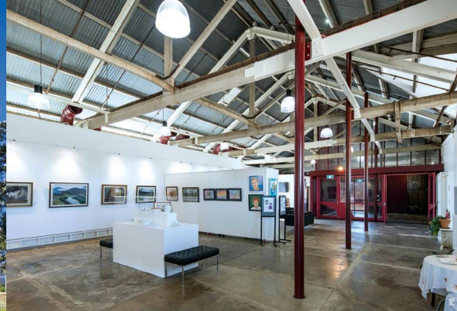
TOP LEFT: The architects have subtly modulated the depth and structure of the roof plane – made from COLORBOND® steel in Apex Apspan 700 profile and Stramit® Corrugated profile, in the colour Manor Red® – which is slimmer above the eaves and thicker above the built envelope
