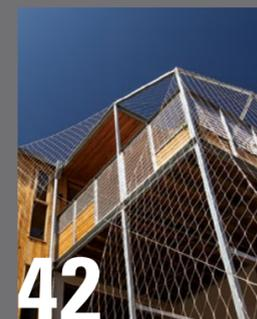
Architect Fiona Winzar has employed a chorus of steel as framing, cladding and shading, to transform a tired former clinker-brick town house
