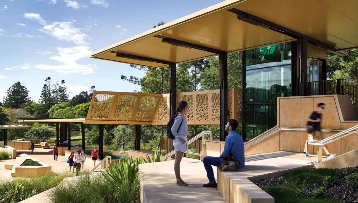
ABOVE: Seven-metre spans of Bondor Equideck® panel made from COLORBOND® steel in the custom Metallic colour Callisto™ create a smooth, uniform finish. A high level of structural steel fabrication creates a bespoke finish that also in-sets custom lighting diffusers
