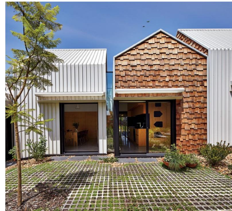
Steel was selected very early on in the process for its ability to provide the material profile which could meet fifth facade aspirations, as well as visually link the six new buildings
