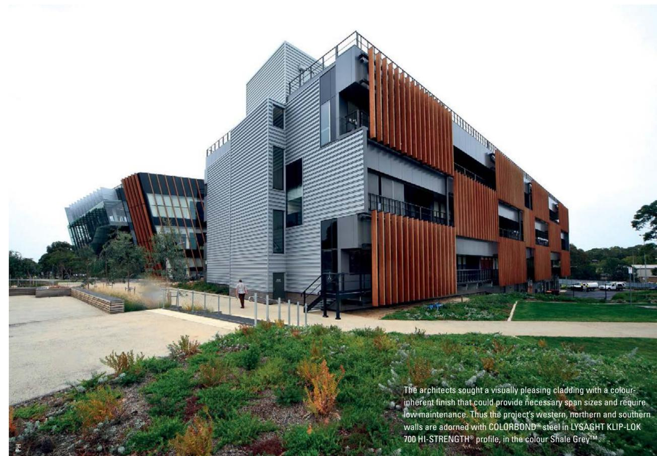
The architects sought a visually pleasing cladding with a colour-inherent finish that could provide necessary span sizes and require low maintenance. Thus the project's western, northern and southern walls are adorned with COLORBOND® steel in LYSAGHT KLIP-LOK 700 HI-STRENGTH® profile, in the colour Shale Grey™.
