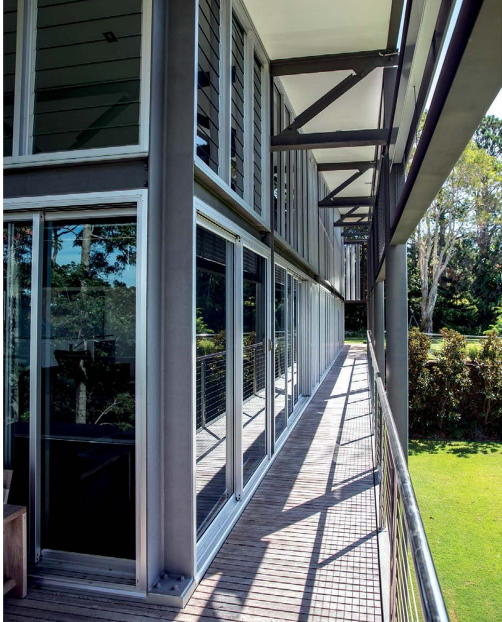
ABOVE: The superstructure was constructed from a variety of RHS, UC, UB, EA, UA, PFC and T beam steel sections and topped with an over-size roof to create a zone through which to run banks of climate-modifying louvres
