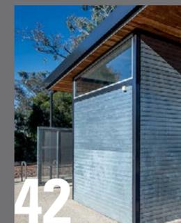
Townsend + Associates Architects sought an economical and tough material to finish the walls of a Canberra toilet block and found it in a material more commonly used for fencing
