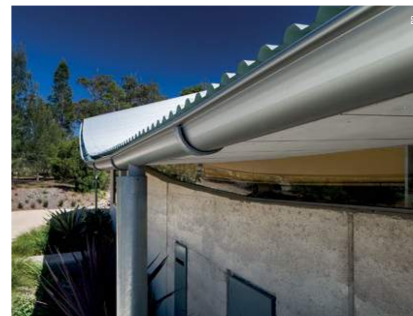
TOP: The slender low profile roof is supported by a structure made from prefabricated 100UC and 200UB steel members which were bolted together on site
