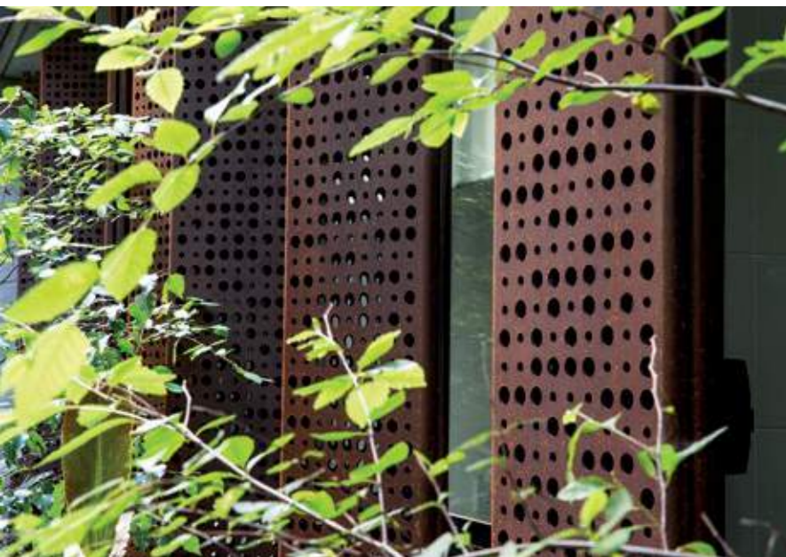
Some of the weathering steel panels are perforated to allow filtered light through to the communal spaces and bedrooms, without compromising privacy
