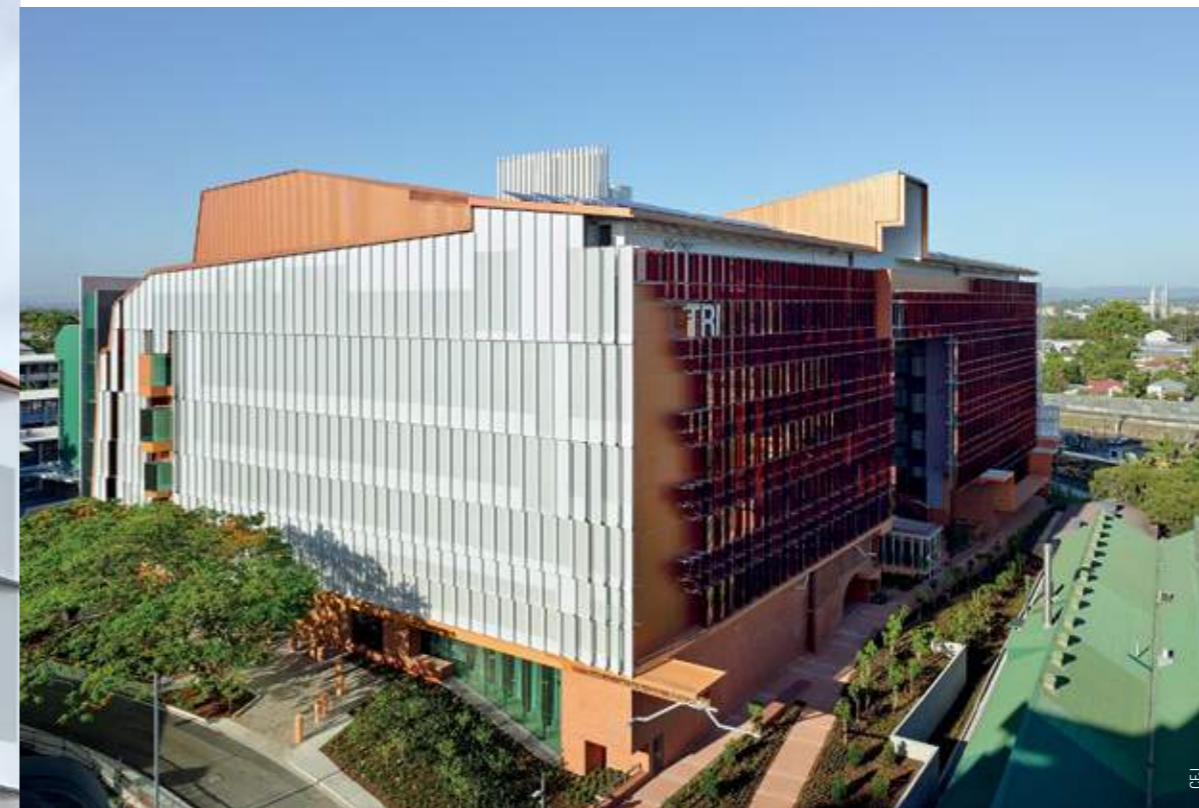
ABOVE: The eastern facade features a sunscreen of perforated aluminium shades clipped to the exterior with galvanised steel framing
