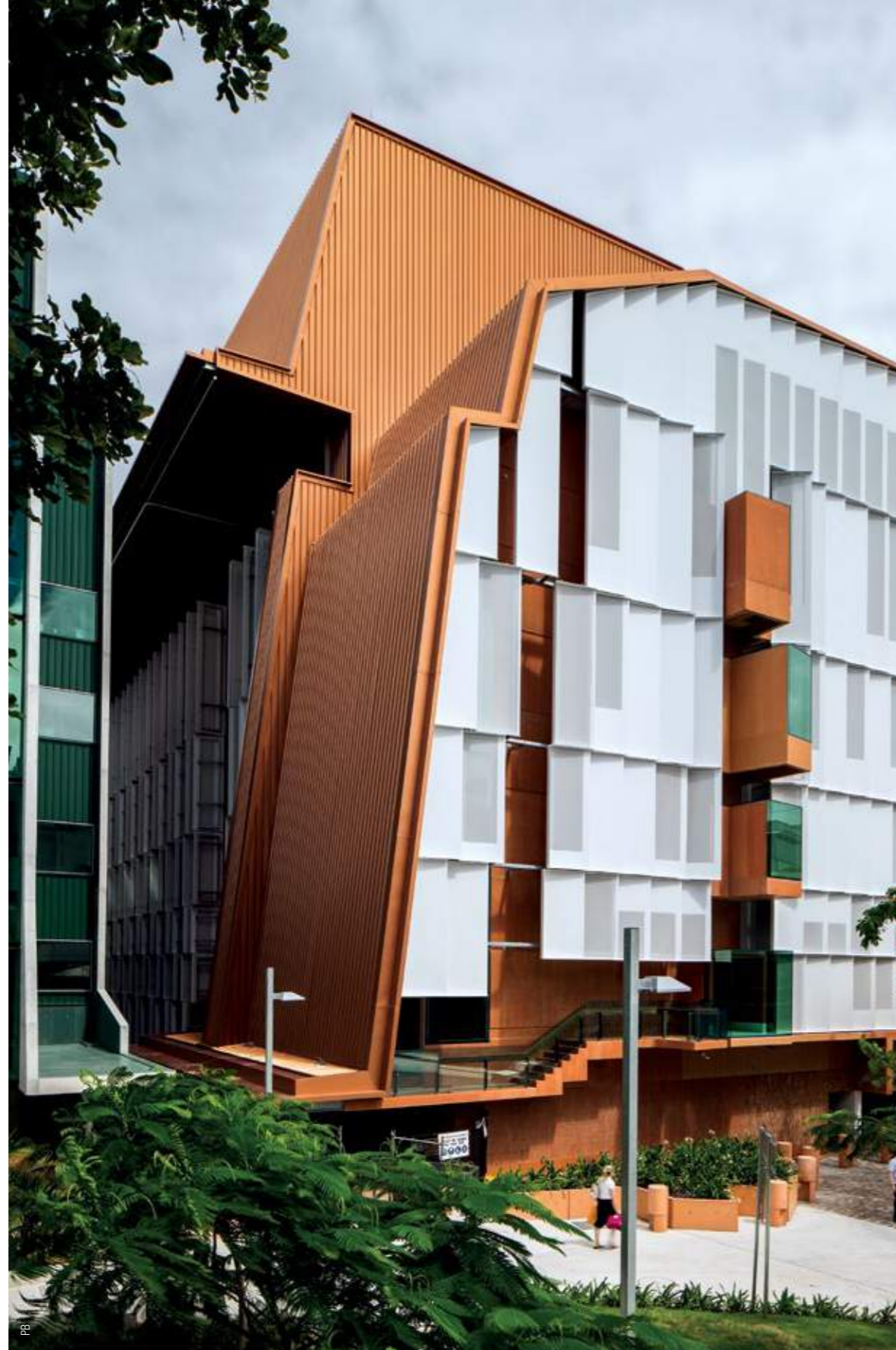
ABOVE: Pedestrian connections enhance access for TRI and hospital campus workers. The wall cladding made from COLORBOND® Metallic steel in the colour Copper Penny, in Stramit Speed Deck Ultra® profile, provides a textural and tonal contrast with the recycled bricks and rose glass
