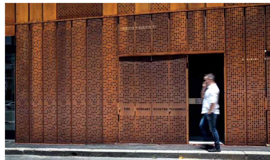
ABOVE A simple gutter made of folded weathering steel directs water away from the doorways to bicycle storage and garbage rooms off Dwyer Street
