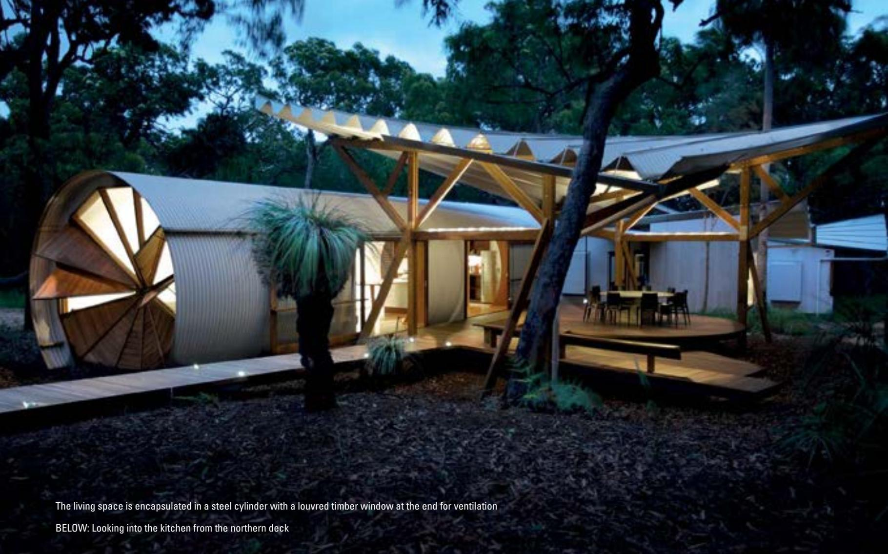
The living space is encapsulated in a steel cylinder with a louvred timber window at the end for ventilation
