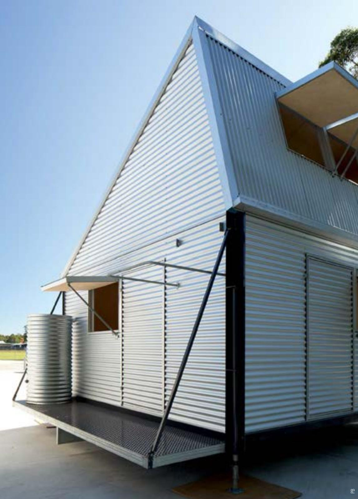
the structure. "In emergency situations the ground isn't going to be properly prepared so the ability to adjust the height of each acrow-prop leg makes them ideally suited to uneven terrain," Carter says.
