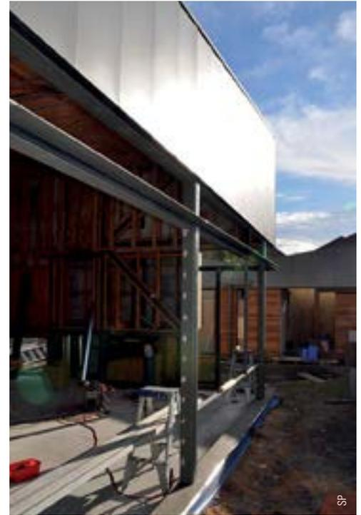
LEFT: The Brighton House, currently under construction, will feature expressed structural steel in the roof form and PFCs along the roof edge to create a folded floating plane, responding to the heavier mass of the original house
