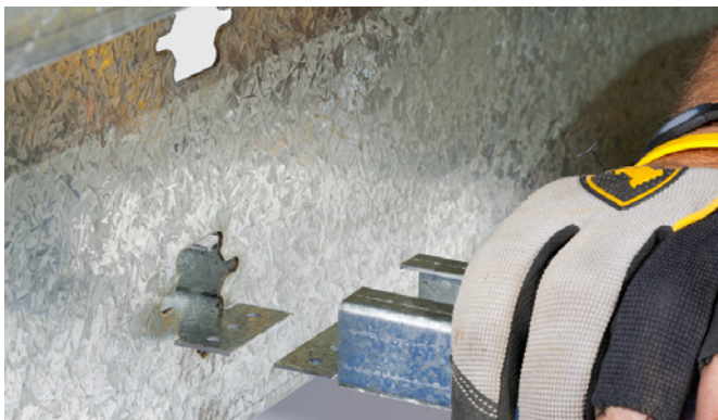
Purlin Keyway - simple roofing screw assembly
