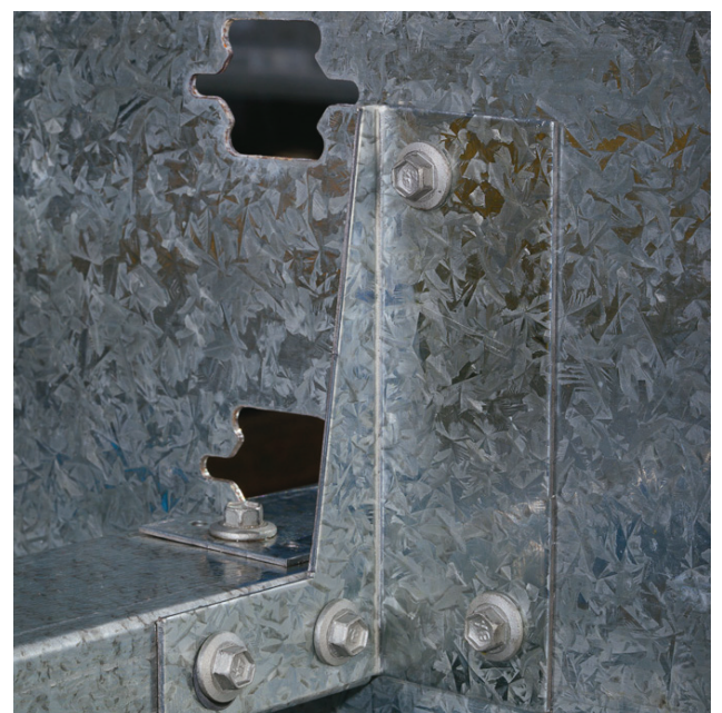
Bridge Bar Stabiliser - prevents purlin 'roll'
