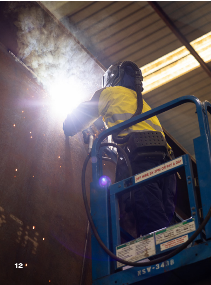
Fitzroy River Bridge featuring welded beams made from REDCOR® weathering steel Kimberley, WA Below: Detail images from fabrication through to installation of various bridge projects across Australia
