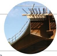
Weathering steels can contribute to improving the sustainability of a structure by avoiding the need to paint (and repaint) structures.
