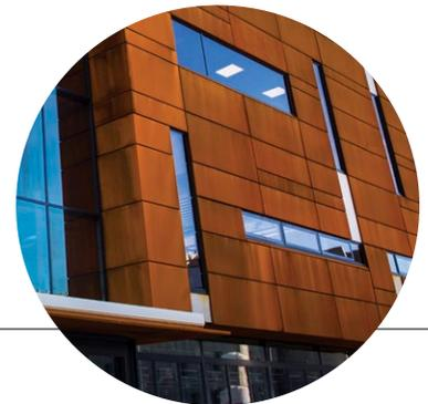
“The cladding made from REDCOR® weathering steel helps identify the main entry to the building and strongly articulates its frontage to the public domain.”
