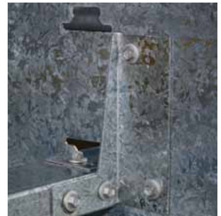
BRIDGE BAR STABILISER Prevents purlin roll
