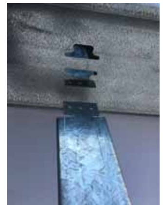
PURLIN KEYWAY Simple roofing screw assembly
