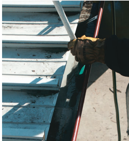
5) Use a soft bristle brush and sweep the dirt out. Rinse again.
