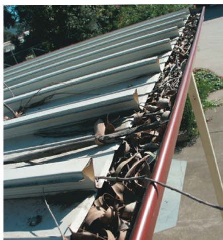
1) A typical suburban gutter clogged with leaf litter prior to cleaning.
