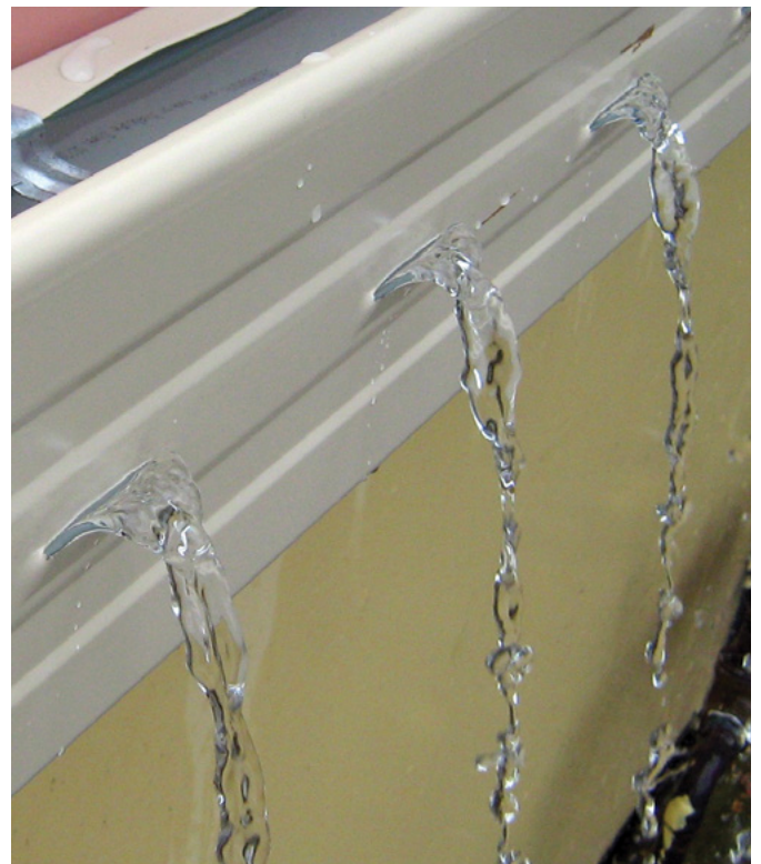
Typical overflow from slotted gutter.
