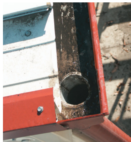
3) When litter is removed, the layer of hardened dirt is revealed below.
