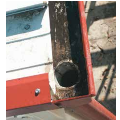
3) When litter is removed, the layer of hardened dirt is revealed below.
