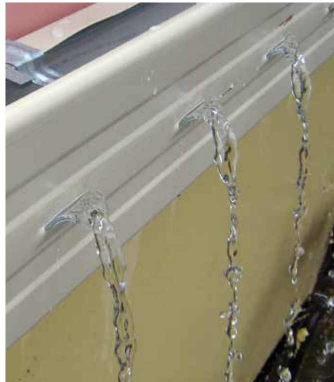
Typical overflow from slotted gutter. (Gutter shown is not available in all areas).
