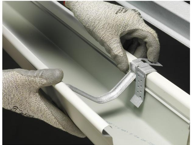
Step 3: Attaching the gutter overstrap
