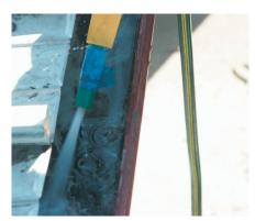
4) Rinse the gutter with water to soften and break up the dirt.
