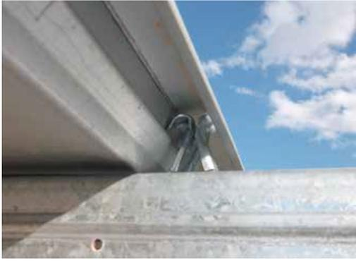
4. Position the tower of the Ampelite Clearslide® HS clip (A) centrally under the Clearslide® HS sheeting, on the support at either end of the translucent sheet. Ensure the Clearslide® HS translucent sheet is square and parallel to the adjacent previously installed KLIP-LOK 700 HI-STRENGTH® cladding.
