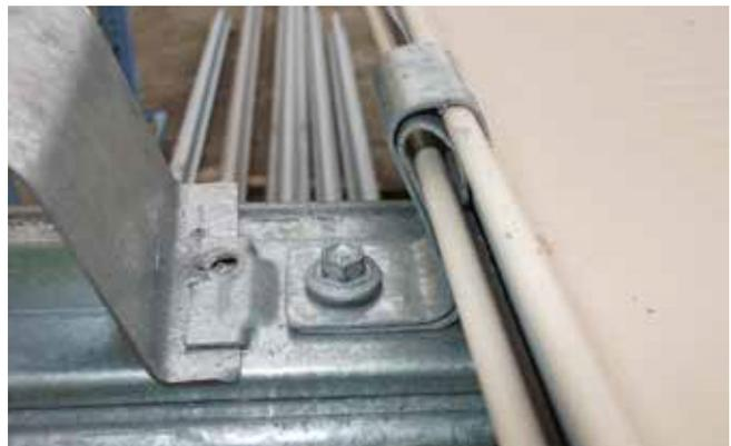
10. At the intersection of the overlap ribs, the LOK-KLIP® joint and the Clearslide® HS sheeting, place a 1200mm (min.) long x 20mm x 19mm slow recovery PVC foam weather strip with adhesive backing on to the top of the lower sheet. Insert 50mm of this foam weather strip inside the void of the overlapping ribs. See Figure 7.
