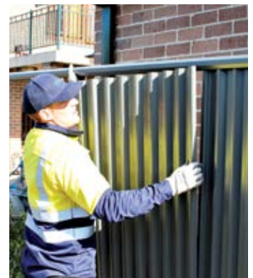
Place 2nd & 3rd sheets into bottom rail, ensuring there is sufficient overlap.
