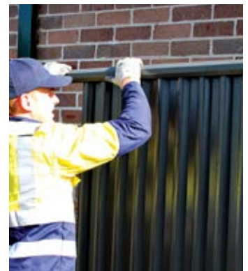
Lift top rail and rotate until all infill sheets slide into rail. Tap top rail down but do not fasten into position yet.
