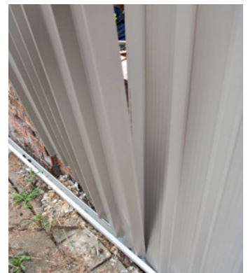
Place 2nd sheet into bottom rail, ensuring there is sufficient overlap.
