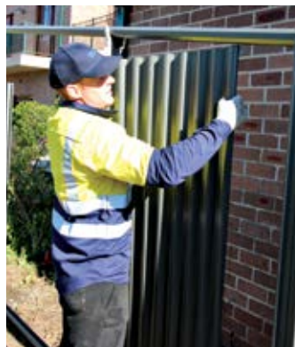
Lifting top rail helps ease 1st sheet into end position.
