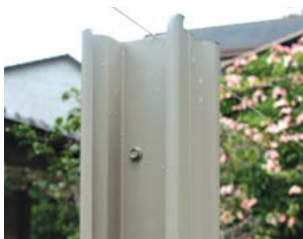
Use stringline to set post heights.
