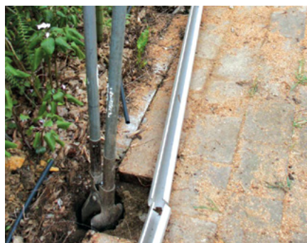
Lay the rails along the string line to determine positions of posts.
