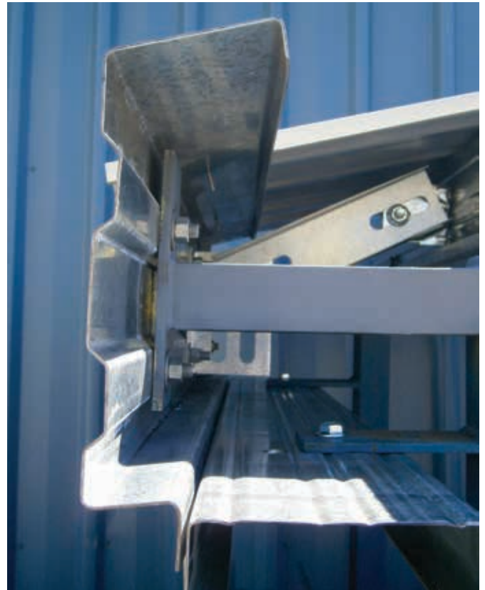
Fascia purlin shown mounted on a building.
