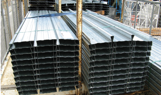
Step 1: Open BONDEK® sheet bundles.
