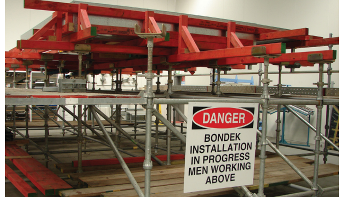
Step 2: Place props if required.
