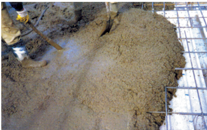
Step 8: Place concrete.
