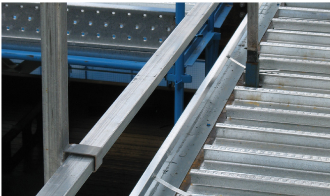
Step 5: Fix steel Edgeform.
