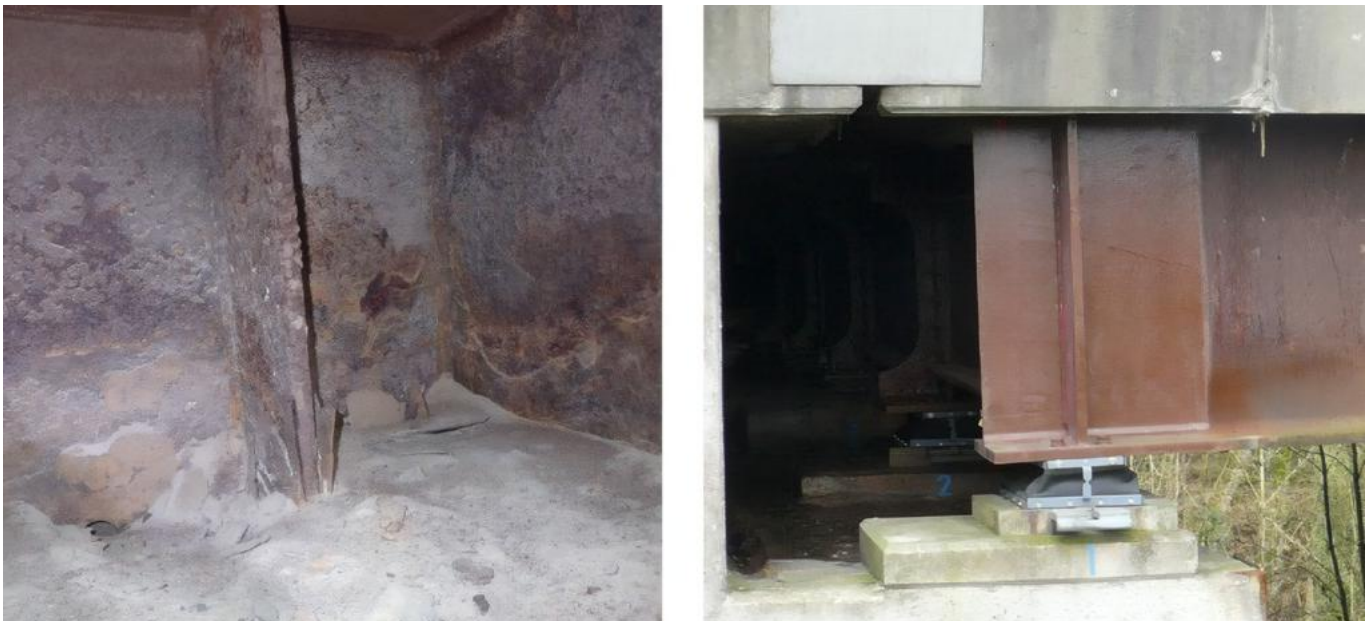
Figure 3-13: Damaged oxide layer due to leaking expansion joint and poor drainage system at the abutment (left) and a local rehabilitation of a damaged area with a subsequent corrosion protection coating
