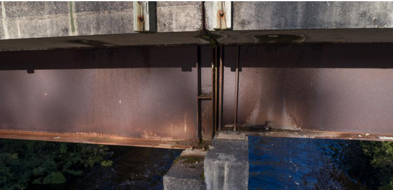
Figure 3-18: Bad detailing of drip plate. Drip plate improperly set at 90°, creating corner for debris accumulation
