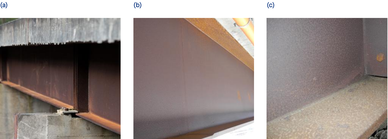
Figure 5-1: Examples of good performing patina
