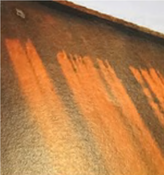
Figure 4-2: Staining from surface markings, not correctly removed
