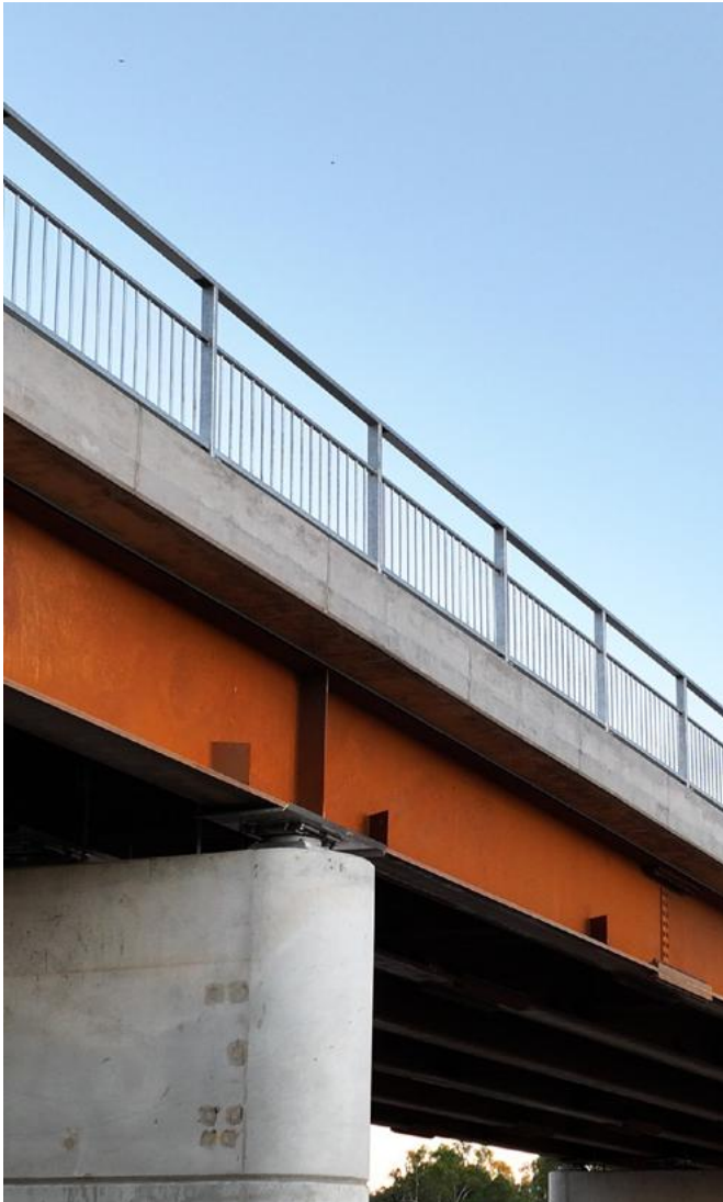
Figure 5-4: Example of a 6 month old patina (left) on Fitzroy River Bridge, WA, and a fully formed patina, after 50 years of service (right) on Frankland River Bridge, Tasmania
