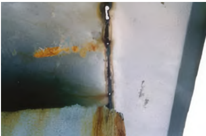
Figure 3-24: Good and bad detailing of a retrofit drip pan – Images courtesy of TxDOT
