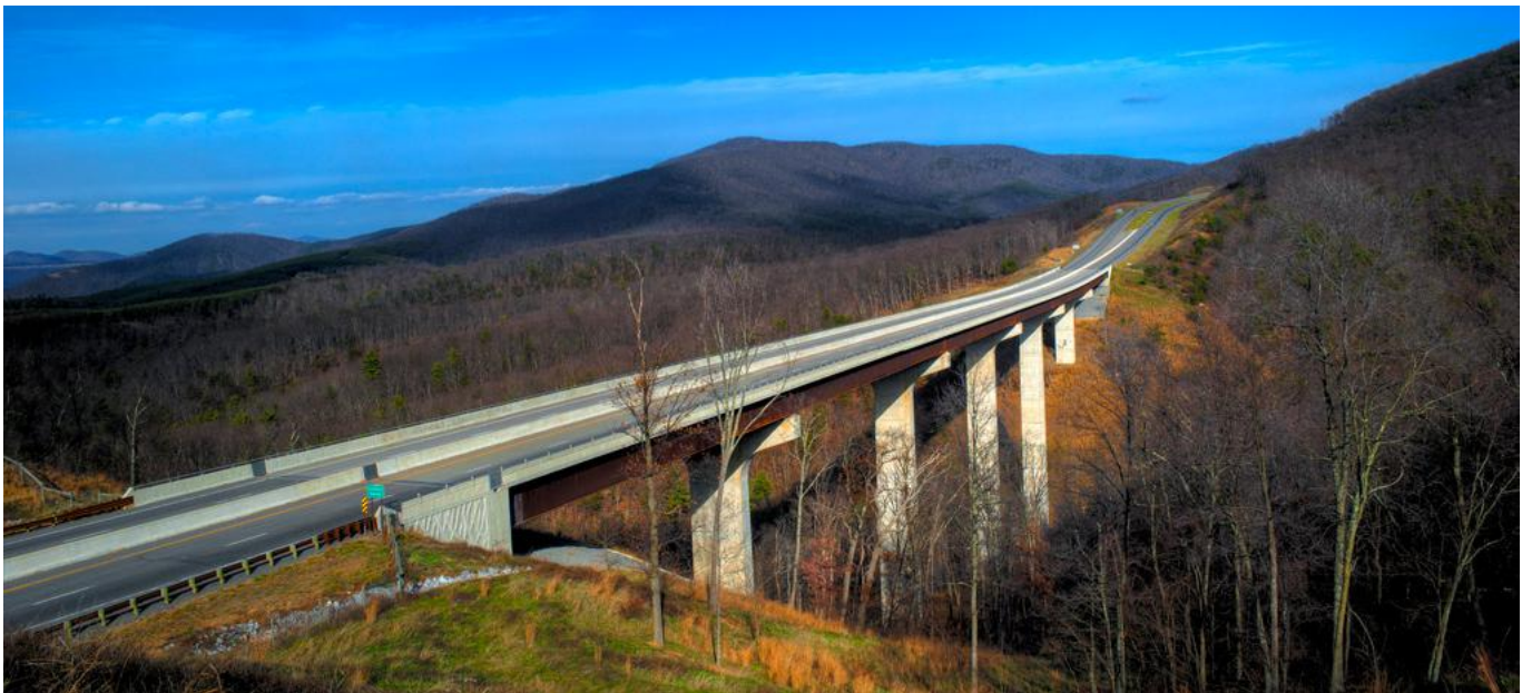
Figure 3-12: Long span “jointless” bridge
