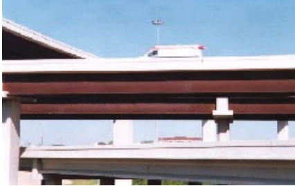
Figure 3.9 Long span “jointless” bridge [image courtesy of the Texas Department of transportation (TxDOT)]
