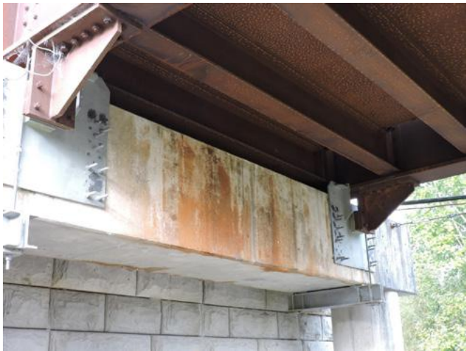
Figure 3-17: Bad detailing (severe staining)
