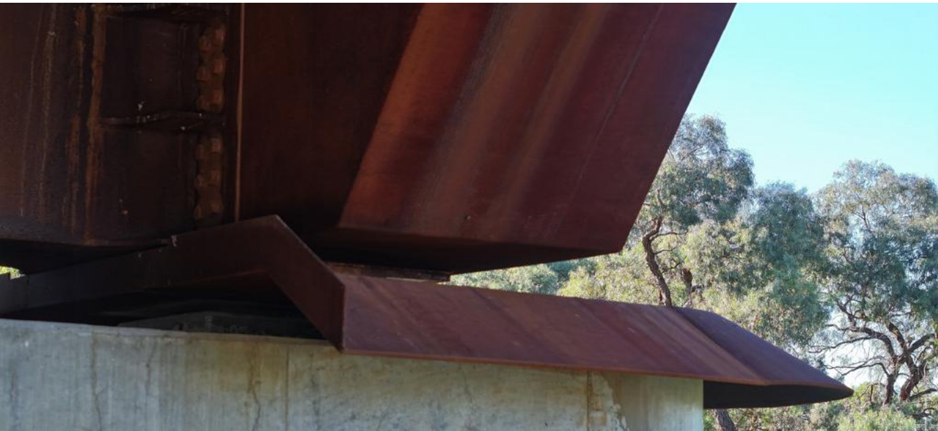
Figure 3-21: Drip pan example below box girder
