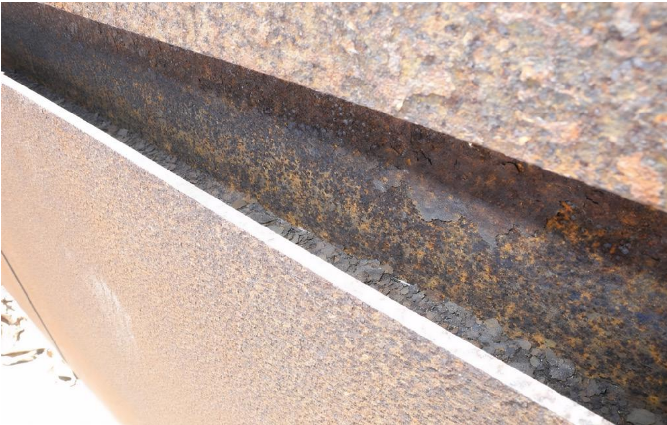
Figure 5-3: Example of granular rust flakes
