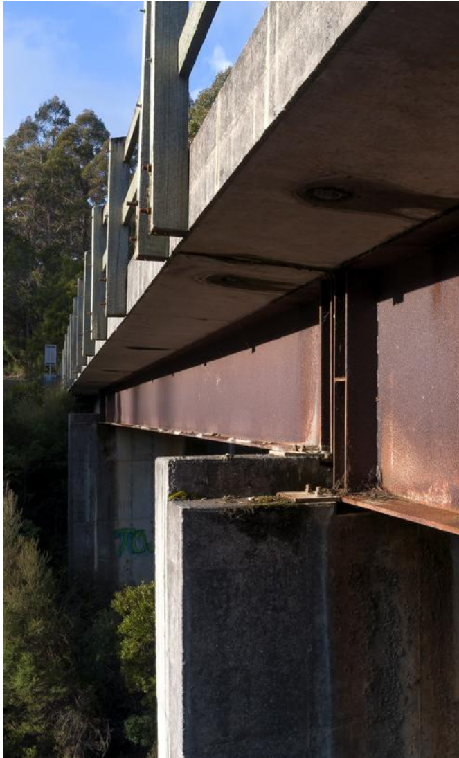
Figure 5-4: Example of a 6 month old patina (left) on Fitzroy River Bridge, WA, and a fully formed patina, after 50 years of service (right) on Frankland River Bridge, Tasmania
