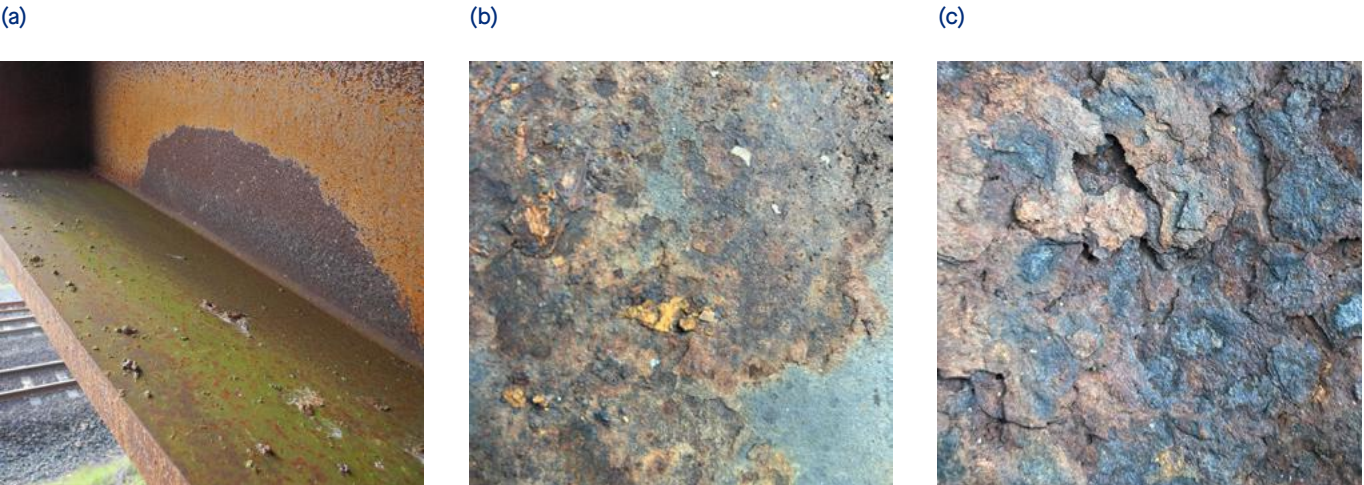
Figure 5-2: Examples of poorly performing patina
