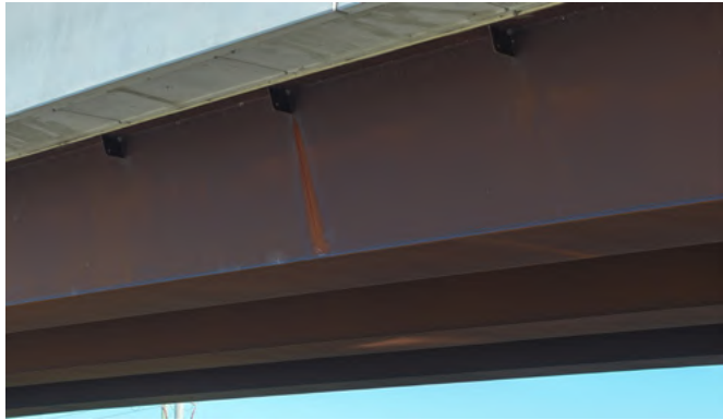
Figure 2-1: REDCOR® weathering steel Patina on Pestells Lane Bridge, Princes Hwy, NSW
