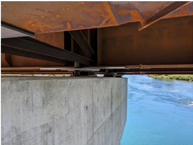
Figure 3-16: Good detailing producing an abutment free of staining
