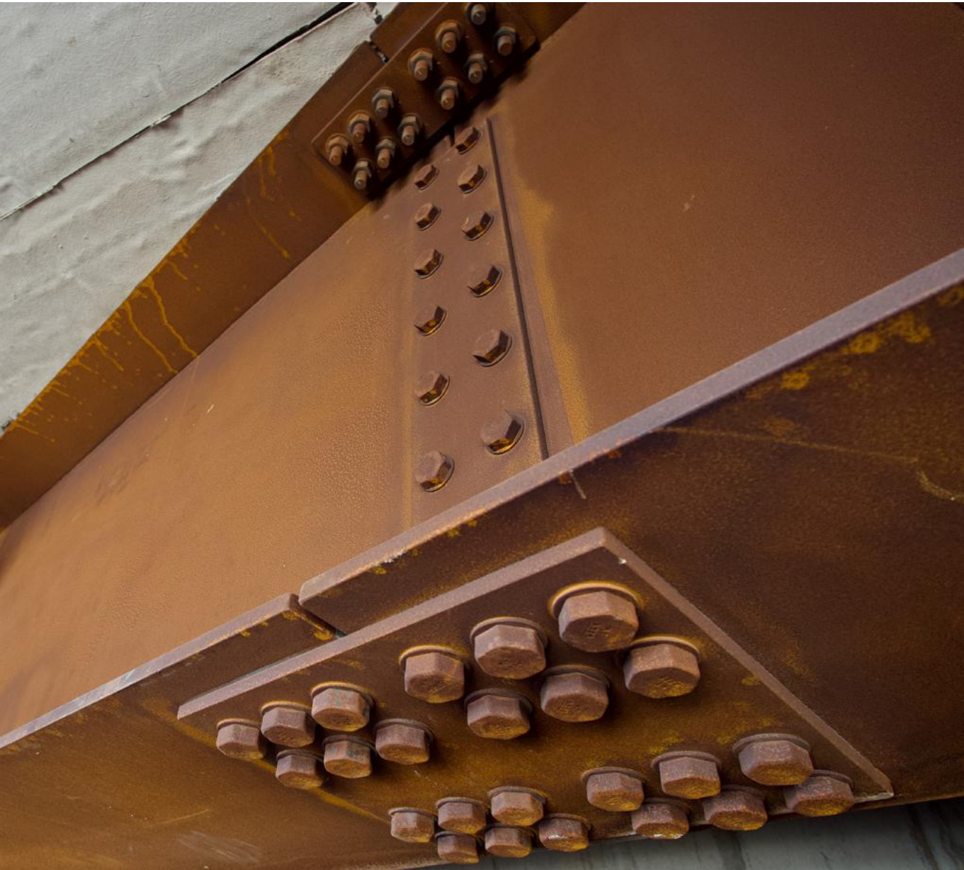
Figure 3-1: Bolted Connection on Sydney Gateway Project SB21, Mascot, NSW
