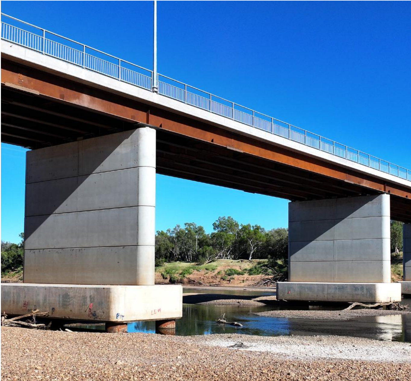
Figure 4-3: Fitzroy River Bridge featuring welded beams made from REDCOR® weathering steel, Kimberley, WA
