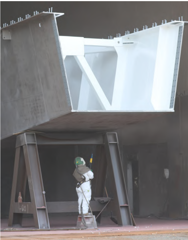
Figure 4-1: Example of surface contamination in the form of mill scale (above) and blasting of the steel surface (below)
