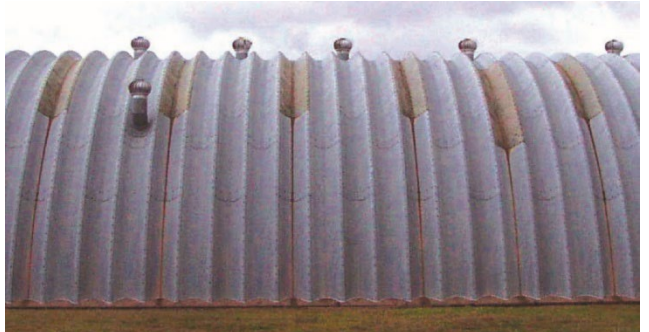
Figure 5: Fibreglass skylights in conjunction with zinc-coated steel sheeting
