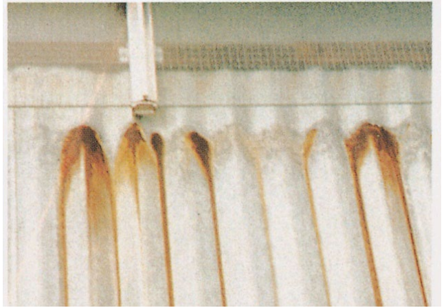
Figure 4: Water flowing from a terracotta roof into zinc-coated steel gutter
