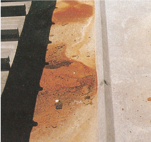
Figure 2: Prepainted zinc-coated steel roofing with zinc-coated steel gutters
