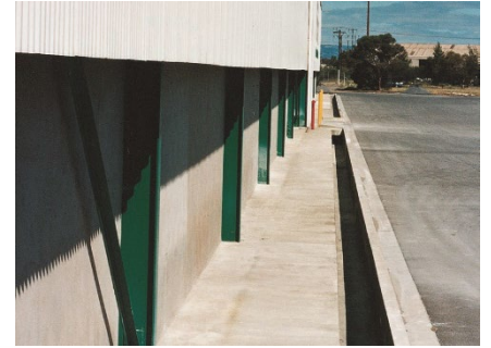
Figure 3: Example of a dwarf wall
