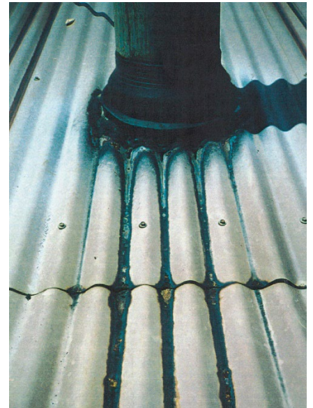
Figure 1: Flue Deposition/Corrosion
