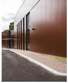
The architects carried out a rigorous process of research and analysis before choosing COLORBOND® Metallic steel in the colour Aries® for the feature cladding, which makes up about 50 per cent of the total cladding.
