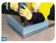
Use a roofing square to fold the stud to 90°, clamp into position and fasten.
