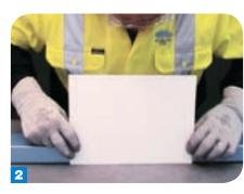
To make your own template, you'll need a thin piece of cardboard about 300mm long. Choose a section of stud that you want to cut, and place the cardboard flush to the edge of the flange on a flat surface.
