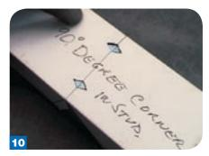
To make the  $90^{\circ}$  corner, you only need to mark a fold line on the web of the stud. Using the diamond holes on the template, align the template fold line with the stud fold line.
