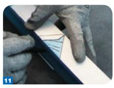
Mark lines onto the flanges ensuring to mark the lap notches under the flange lips. Then, notch out material, and safely dispose or recycle.
